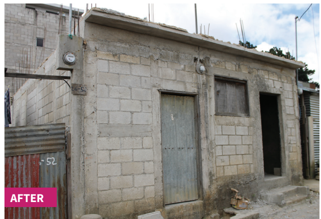
Added and strengthened interior walls; new reinforced concrete slab roof
