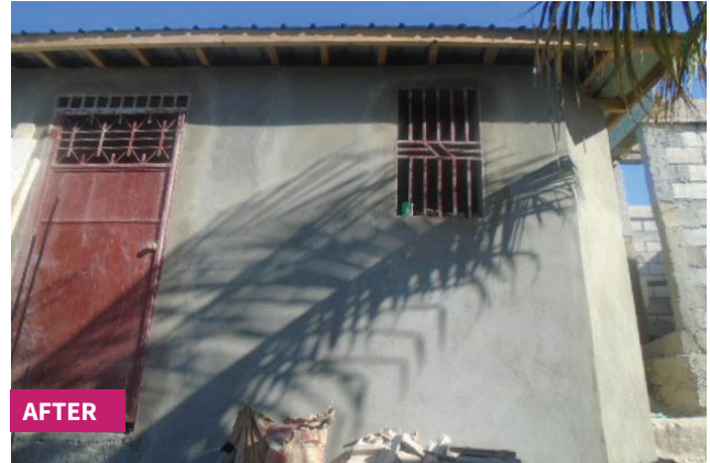
New ring beam, repaired damaged wall, added plaster, and new roof
