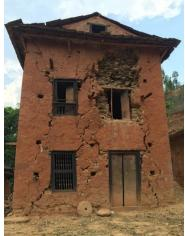
Fig. 9. Short wall damage
