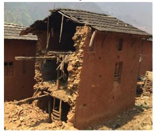
Fig. 11. A damaged house in Sindhupalchowk where the entire short wall is collapsed but the house is still standing
