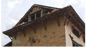
Fig. 8. Gable wall damage after earthquake
