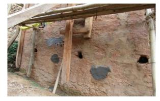
Fig. 13. Installed through wall concrete connections
