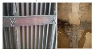
Fig. 24. Showing GI wires, threaded rods and metal plates used in the construction
