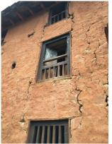
Fig. 10. Vertical cracks observed at floor level in a typical SMM house
