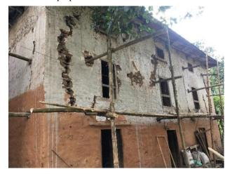
Fig. 26. Damaged house prior to retrofitting
