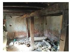
Fig. 5. Wooden posts, Girder beam and joists in a typical SMM house in Kavrepalanchowk
