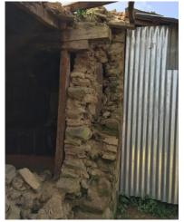
Fig. 7. Cross section of a SMM House showing the dual layer of stones
