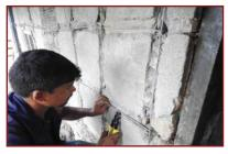
Install horizontal wires on both faces of walls in the portions not covered by the belts.
