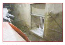
5. Mark Sill belt under the window if sill is 600mm (2') or higher. Otherwise at approximately 900mm (3') from the bottom of Lintle Belt or close to mid height mark the belt. If window is close to the floor, discontinue the belt or continue a smaller width belt under the window.
