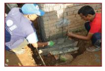
**10.** Pour 1:1.5:3 concrete continuously rodding to prevent cavities in concrete. Cure concrete for 15 days.
