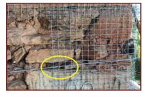
**4.** When a wire goes over and across the Splints it should be tied to Splint at minimum 3 points with 1mm GI binding wires.
