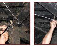
1. Install GI wire diagonal ties 2. Use carpenter's hammer to pull the wire taut while installing on underside of the roof with the wire. After installing all 4-2mm GI wires twist them together
