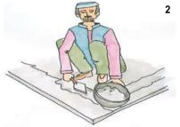
2. Apply 1:3 cement - fine sand mortar over the crack, and cure for 15 days.
