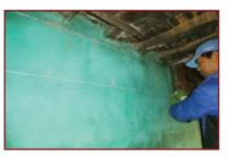
3. With top edge of belt marked, next mark the bottom line of the belt on all four walls to get the desired width 300mm of the belt
