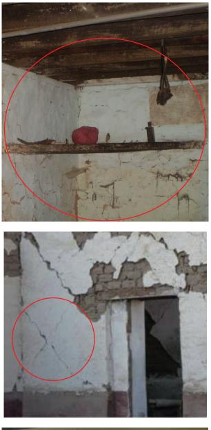
C1.1 Low strength masonry : Stone Masonry in Mud mortar
