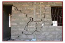
Grade 3 cracks between opening
