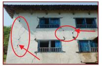
Grade 3 cracks in plastered wall
