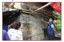
**3.** Install the prepared WWM on the raked and clean wall surface where the cross links are pushed in and anchor it with nails first.
