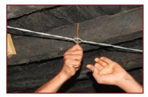
**6.** Pre-tension each Tie by pulling at the time of installation followed by twisting. Excessive twisting can break the wires.
