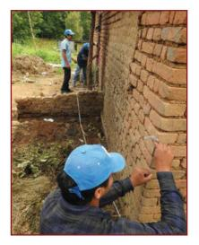
7. Using the tube level mark the top and bottom line of the belt on the outside walls, ensuring same level as on inside walls.
