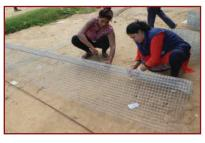
1. Make WWM straps 800mm wide for L and 400mm wide for T junction for full wall height with 450mm extra for starting below plinth level.
