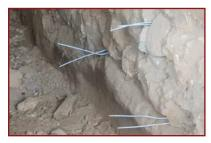
2. Insert cross-links in holes. Be careful of cross-links protruding out and protect eyes from injury.
