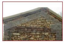
**18.** Install gable belt with its top edge approximately 100-150 mm below the top edge of gable wall.
