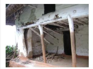
Diaphragm failure: Lack of proper connection of diaphragm: floor/ roof with the wall result in failure of floor/roof.
