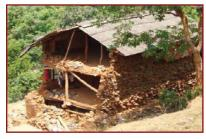
Parts of wall or full wall collapsed because of poor wall to wall connection or the walls were too long or too high
