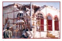
Cracked arcade being restored stone by stone.
