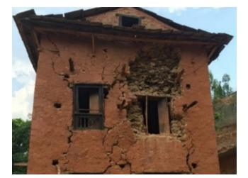
Figure 3: Short wall out-of-plane damage in SMM building
