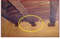
Sliding of timber joists sitting on bearing stones projecting out from walls.
