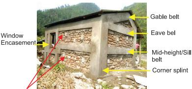
Horizontal and Vertical CR wires are to be installed in the spaces left uncovered by the belts and splints.
