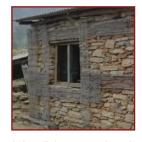
2. Install the prepared mesh in right location with right overlap with Lintle & Mid-Height Belts.
