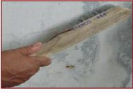
2. Clean crack with wire brush to remove all loose materials including dust.
