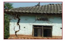
Vertical cracks developed at corners because poor wall to wall connection.
