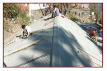
Nails being replaced by 'J' hooks to anchor tin sheets to purlins.
