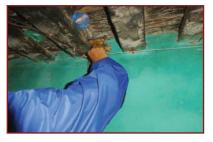
1. Mark the top line of Lintle belt just under the floor joists on an inside wall, while ensuring that it clears the bottom of most of the floor joists. Disregard the bottom of the beam that supports the floor joists which is significantly lower.
