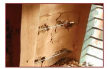
5. When a wire is interrupted by a wall opening, wrap it around the jamb to continue on to the other face of wall.
