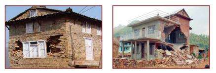
Typically, this type of damage is most commonly interpreted as total loss or total collapse, and is considered fit for reconstruction. However depending upon the spread of the damage and intensity, building could be restored on the case to case basis. Only those engineers with understanding of structures and damage would be able to advise on repair, restoration and retrofitting of buildings with partial collapse.
