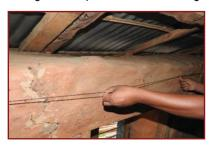
**10.** Mark the top line of Eave belt with string 150mm (6") below top of the wall. Follow the same on all four walls inside and out side using tube level.
