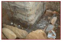
9. Install form work not exceeding 150mm in width from the steel cage to prevent wastage of concrete.
