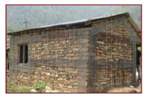
**6.** Vertical and horizontal CR wires in the open spaces between belts and splints.
