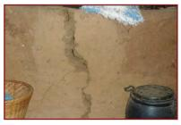
4. If the structure has mud mortar or mud plaster then seal the crack with mud
