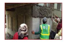
**16.** While still wet, apply neat cement slurry followed by first coat of cement: coarse sand (1:3) plaster of 12mm (0.5") thickness.
