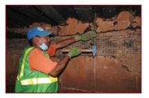
**3.** Mark the exact location of the vertical wires on the underside of ceiling. Drill hole through the floor.
