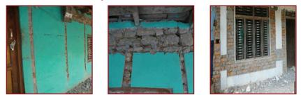
Rake all the mortar joints to the depth of 12mm (1/2") by hand using chisel. Clean the surface with wire brush and water.
