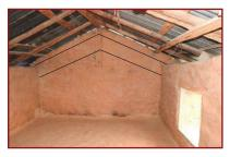
**13.** Mark Gable belt 150mm (6") below the top edge of the gable wall. while ensuring the proper connection with attic wall Eave belt.
