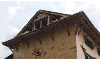
Figure 2: Damaged gable wall in an SMM house
