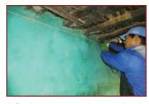
2. Consider this level as the datum. Use the tube level to get the correct level and mark the top line of the belt on all four walls with cotton string. The belt alignment can be above or below this datum depending upon the obstructions like beam, window etc.
