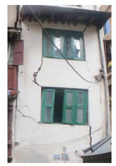
C.2.2 Low strength masonry : Brick masonry in mud mortar
