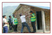
4. With the tube level follow the same level and mark the top and bottom line of the belt on the outside faces of walls.
