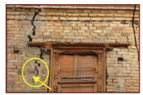
Grade 3 cracks in un-plastered wall
