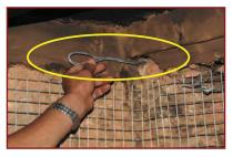
1. Install special cross-link made of 2-2mm wires folded at mid-length to make a loop at one end in four corners of each room through masonry walls .
