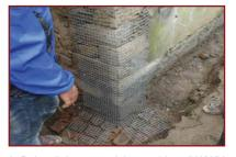
3. Rake all the mortar joints and Install WWM splint starting from 450 mm below plinth level and continue through to the top of the wall at roof level.
