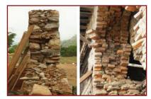
Faces of Stone and brick walls separate when Headers are not provided or are not enough
