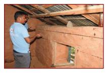
**11.** Measure the width of the Eave belt from top line of the belt and mark bottom line of the belt with the help of the tube level.
