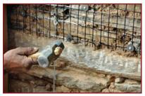
**4.** Hammer in 100-150mm (4"- 6") long masonry nails in mortar joints in zig-zag manner at 300mm spacing to anchor the belt securely to the wall.
