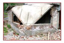
Consisting of wide crack with a portion of the slab bent resulting in bending and exposing of reinforcing bars.
