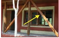
Alternatively, diagonal wooden bracings between column can be installed if space permits.
