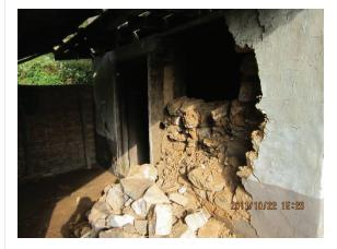
Collapse of wall: When the out of plane bending capacity of wall is exceeded, partial or complete collapse of wall happens.
