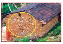
Dismantle the cracked walls further in step like manner all the way from ground level, while propping up the roof and floor. Rebuild walls to connect well with adjacent walls, floor and roof
