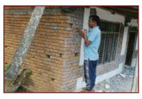
2. Install shear connectors a day before the splint installation. Continue to cure until splint is plastered. Exercise care not to exert too much force on shear connector while splint installation.
