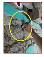
7. Insert small stones or stone chips below and above the cross links using little mud mortar for closing the hole.
