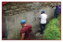
2. Follow the same process and mark vertical lines on all walls between the splints for vertical CR wires on both faces of all walls. Remember vertical CR wires are not to be located on any WWM splint or encasement. They can go over horizontal belts.
