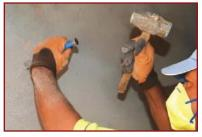
1. Make 'V' notch along the crack to broaden the mouth of crack. Do this carefully so as not to damage the wall.
