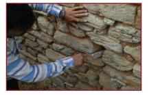
**2.** Make small hole approx. 100mm X100mm (4"x4") and 250mm (10") deep by removing stone at desired location. Clean the hole with wire brush and water.
