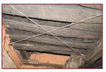
**4.** Install in-plane diagonal tie in 'X' configuration made of 4-2mm GI wires in each tie pulling wires tightly .
