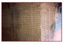
**11.** To ensure continuity of WWM with upper storey, at the top end under the ceiling, install 4-4mm wires on each leg with 600mm overlap plus 150mm long hook, and extend up to storey above
