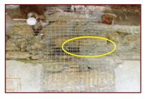
**4.** Use 100-150mm long nails with washers driven in open joints at 300mm spacing to anchor WWM to wall
