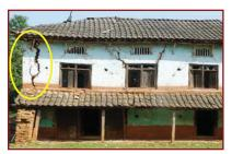
Out of plumb detached wall to be removed along with adjacent walls in stepped manner, and rebuilt to connect well with other walls, timber floor and roof. Cracks in window corners are to be filled with mud and spliced.
