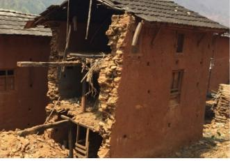
Figure 4: Collapsed gable wall
