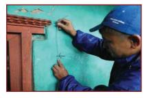
2. Simultaneously start marking the opening encasement on the sides of openings. Use plumb bob and mark vertical lines. Follow the same lines on both faces of the wall. Once lines are marked, mark the location of cross links as per the specification.
