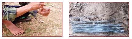
Make cross-links by twisting together two 2mm GI wires 150mm (6") longer than the wall thickness. Leave 65 to 75mm (2.5" to 3") long unequal ends straight and untwisted at both ends.
