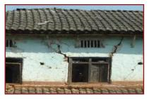
Large diagonal cracks developed at the door and window because of the absence of a band at lintle level.
