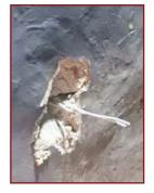
**6.** Make sure open ends of cross-links protrude out from the wall on both faces.
