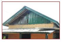
**19.** Alternatively replace masonry gable with GI sheet or timber on timber frame.
