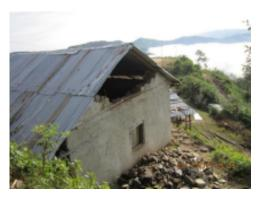
Figure 5: Attic wall out-of-plane damage (Photo credit: NRA)
