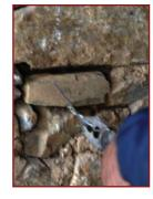
**9.** When pulled, cross-links should not come out without prying out the wedged chips.
