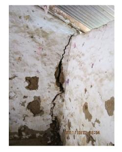
Corner Separation: The lack of proper connection between the orthogonal walls result in Corner separation
