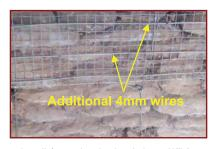
7. Install 4mm wires having 150mm (6") long hook at their ends using 1mm GI binding wires on the WWM belt as required per specifications
