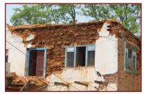
Delamination of a thick brick wall
