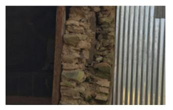
Figure 1: Cross section of a damaged SMM house showing the dual layer of stones (Photo credit: NRA)
