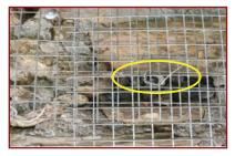
5. Using binding wires at minimum of two places secure vertical splints to shear connectors anchored in the wall.
