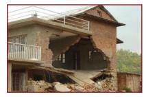
Floor collapse because of collapse of wall and poor floor to wall bonding.
