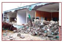
Undamaged RC slab on severely damaged wall
