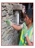
**5.** Insert cross-links in the holes at pre-dermined location on walls.
