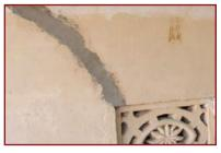
3. If structure has cement mortar and/or cement plaster then seal crack with 1:3 cement mortar after wetting the crack surface and cure it for minimum 7 days.
