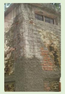
G I wire mesh anchored R C splint
