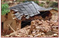
Collapsed roof due to collapsed walls
