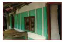
**18.** Finish belts and splints as desired. All vertical and horizontal wires may be covered with 2"(50mm) wide strip of cement plaster or can be left exposed.
