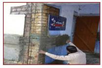
Full height wall to wall separation being rectified with WWM corner splint and additional straps.
