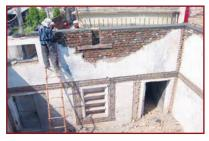
Damaged brick masonry wall being rebuilt to reinstall RC slab on it.
