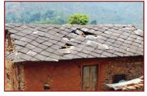
Damaged roof structure and dislodged slate / roof tiles
