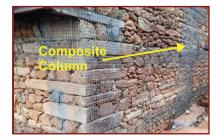
8. When belt length if greater than 5m then install Composite Column as per specifications at the mid-lenght of belt.
