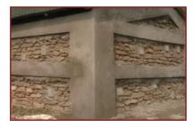
**12.** Cover splints with 1:3 cement - coarse sand plaster in two coats exactly as is done in the belt and cure for 15 days.
