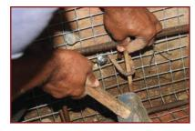
**8.** Anchor the cage to the wall with 6mm U shaped anchors 150mm long hammered in to the masonry joints to hold down the reinforcement tightly.
