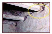
Sliding out of timber joists sitting on walls
