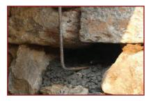
3. Fill bottom half of hole with concrete (1:1.5:3) and place 'L" shaped rod over it with the hook end inside the wall.
