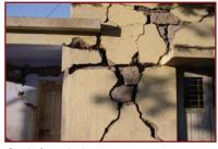
Grade 3 cracks in masonry
