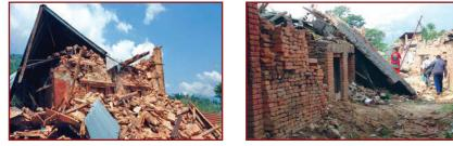
Total collapse of stone and brick masonry houses
