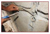
2. Anchor the cross-link with a 10mm diameter 300mm long bar installed against the outer face of the wall.
