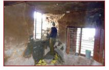
Badly damaged stone masonry wall dismantled and being rebuilt accompanied by a new window.
