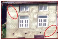
Exposed masonry wall having Grade 2 cracks
