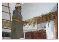
**15.** Splash the exposed wall surface with water to remove all the dust as also to make it moist.
