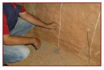
**4.** Using plumb-bob and cotton string mark the alignment of wires in the upper story. Continue up to attic in the same manner.
