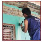
Use electric grinder or chisel and cut the plaster precisely within the area marked for the measure to prevent excessive plaster removal.
