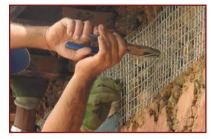
6. Pull out the cross-link ends in such a way that they catch at least two wires of WWM and twist them three times max to tightly anchor the mesh.
