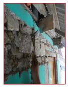
8. Chips must be hammered in strongly to ensure that they lock the stones around them.
