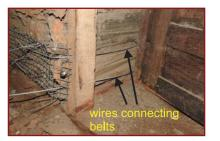
**12.** At the opening jamb install 3-4mm wires connecting belt on both faces of wall with 300mm overlap on faces.
