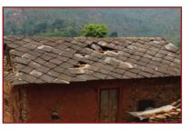
Roof damage because of degraded timber and dislodged slate.
