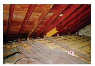
R.4.1 view inside the attic showing the rafters and the absence of collar beams and joist connections to the rafters
