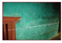
6. Mark the top and bottom line for this belt measuring from the top edge of the Lintle belt. Do not measure from any other point. Use tube level to ensure the right level of the belt along its full alignment.
