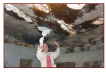
Spalled concrete removed, rusted bars cleaned and coated with anti-rust chemical, bonding agent applied and finished with micro-concrete.
