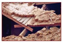
Breaking of floor joists
