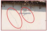
Grade 2 cracks in Cement plastered wall
