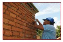
**1.** Start marking the vertical splints at 'L' and 'T' wall to wall junctions. This is installed only on outer face of walls. Use plumb bob for marking vertical lines. Once lines are marked, mark the location of shear anchors as per the specification.
