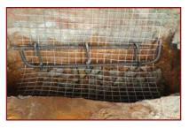
7. Place 10mm dia steel bar cage with weld mesh end projecting out 150mm at the bottom. All hooks of the cage must be bent away from the wall.
