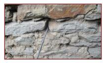
3. The holes shall be just large enough for inserting the cross links through full thickness of the wall.
