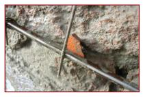
**5.** Provide 15mm (0.5") thick spacers of any suitable material between the wall surface and the mesh to ensure full encasement in plaster.
