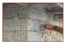
**6.** Where splint overlaps with belt they are tied together with binding wires at 5 points.
