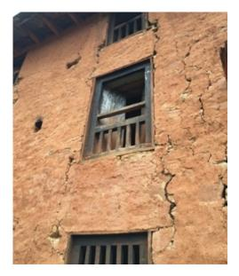
Figure 6: Diaphragm deficiency (Photo credit: NRA)
