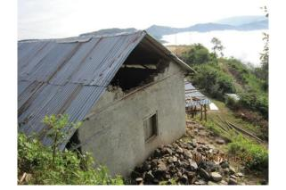
Failure of Gable wall: Lack of proper anchorage of gable wall with the roof results into failure of gable wall. This is the most common type of failure pattern in masonry buildings.
