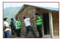
**15.** For accuracy use tube level to match inside and outside levels
