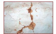
Grade 2 cracks in wall with mud plaster
