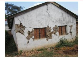
Diagonal Cracks: Diagonal cracks on the walls are the result of in plane bending and shear force. When the in plane bending and shear capacity of the walls are exceeded, such diagonal X cracks are formed.
