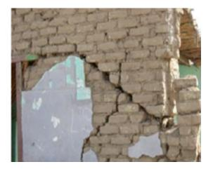
Figure 7: In-plane damage in wall (Photo credit: NRA)
