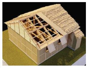
R.3.3 Bracing missing in inclined roof
