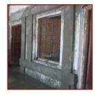
**3.** Plaster encasement using cement mortar in two coats as described earlier.
