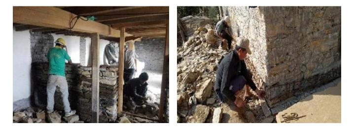
Figure 21: Ongoing architectural modification work Figure 22: Mason preparing foundation for lateral tie on construction of wing walls during retrofitting of beam below the plinth level for tying up reinforcements house in Dolakha
