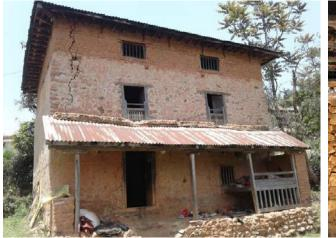
Figure 1: Typical 2.5-storey SMM building (Photo credit: UNOPS, Build Change, BBC Media Action Consortium)
