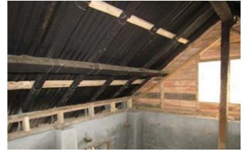
Figure 15: Improvement of existing timber connection (Photo credit: UNOPS, Build Change, BBC Media Action Consortium)
