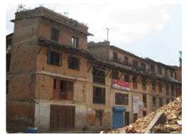
Figure 3: Typical brick in mud mortar house (Photo credit: Build Change)
