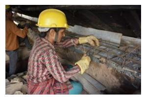
**Figure 52: Participant constructing ring beam at ongoing training on strong back** (Photo credit: UNOPS, Build Change, BBC Media Action Consortium)
