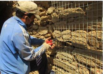
Figure 23: A pair of masons fixing vertical and Figure 24: Anchoring inner and outer mesh of GI wires horizontal strips of welded GI wire mesh as splints and bandages during retrofitting in Dolakha
