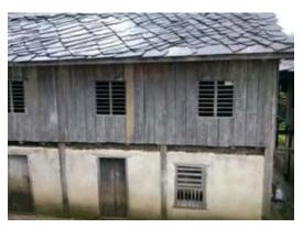
**Figure 6: Typical timber frame structure** (Photo credit: UNOPS, Build Change, BBC Media Action Consortium)
