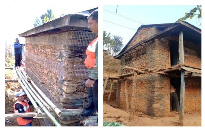
Figure 29: Securing the "bandages" horizontally on walls
