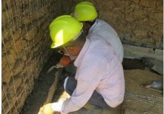
Figure 25: Preparing wire mesh using GI wires and Figure 26: Concreting of foundation tie beam after anchoring to the wall to prevent local failure in stone completion and anchorage of reinforcements masonry building
