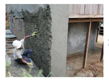
Figure 27: Plastering of surface after completion of all retrofitting works
