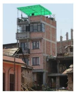
Figure 7: Typical reinforced concrete frame building with masonry infill (Photo credit: Build Change)
