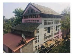
Figure 28: Example of CR integrated splint and bandage technology (Photo credit: UNDP/ Government of India funded Nepal Housing Reconstruction Project in Gorkha)
