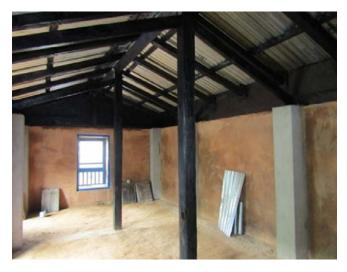
Figure 10: House retrofitted using the strong back approach
