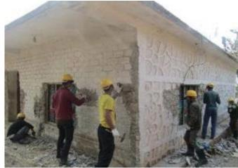
Figure 19: Scaffolding and props seen around a Figure 20: Trainee masons working on removal of cement stone-mud masonry house undergoing retrofitting in plaster and surface preparation of house undergoing retrofitting
