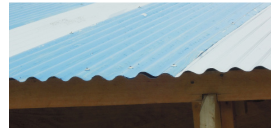
Insufficient roof nails
