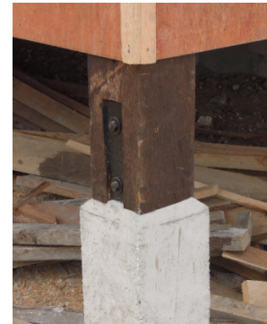
Connected with plate or strap embedded into concrete
