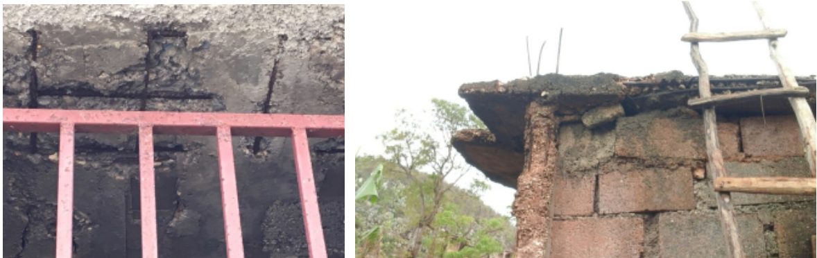
Figure 41 Exposed rebars and insufficient thickness of two slabs
