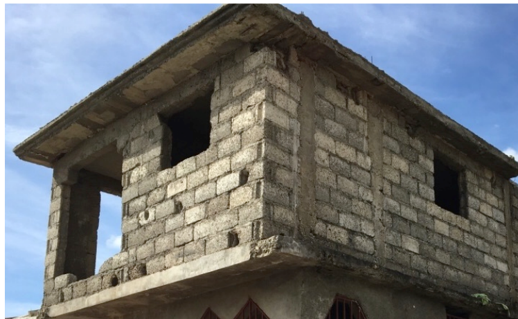
Figure 19 Reinforced concrete slab roof
