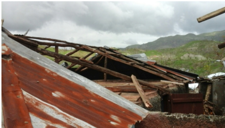
Figure 37 Rusted metal sheet insufficiently nailed to the roof structure
