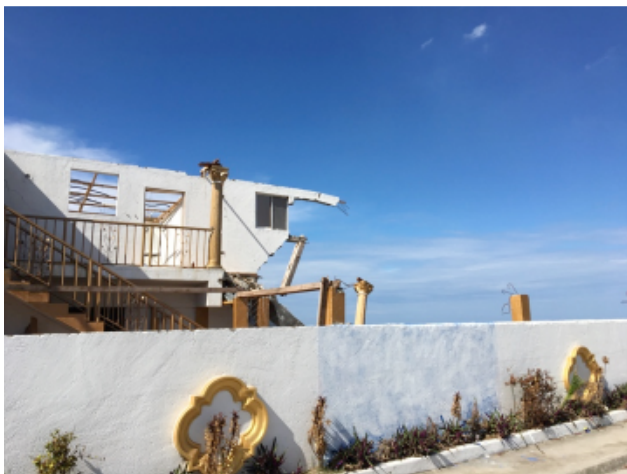
Figure 55 Left: Collapsed hotel in Port Salut due to the storm surge Right: Hotel not damaged but flooded up to the 1m above the first level
