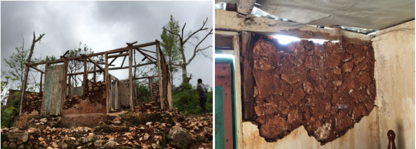
Figure 30 Left: Cracking of the infill Right: Partial wood diagonal bracing in masonry wall infill
