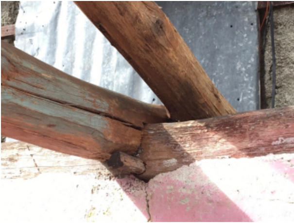
Figure 39 Left: Roof system-to-top plate connection Right: Column-to-top plate connection
