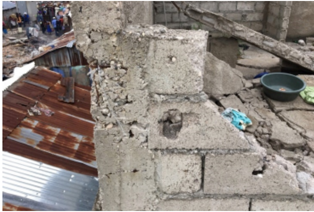
Figure 27 Left: Wall collapse due to lack of tothing and intermediate beam Right: Tall wall collapsed
