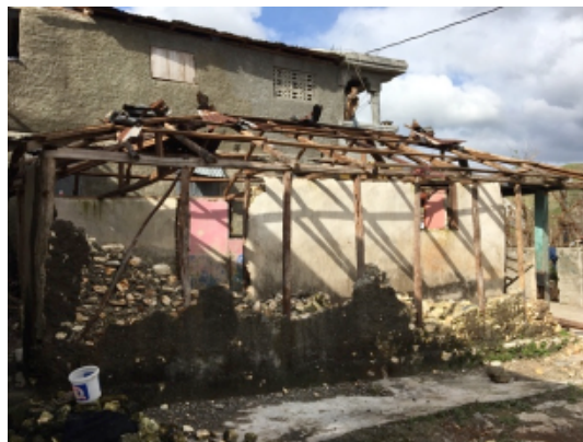
Figure 31 Out of plane failure of masonry infill
