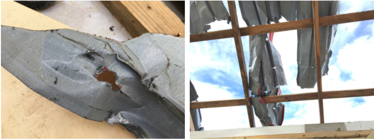
Figure 38 Left: Screw and washer hole on a metal sheet Right: metal sheet torn apart due to insufficient thickness of the sheet
