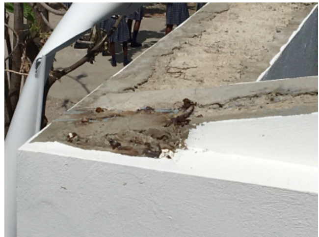
Figure 48 Failure of the welded connection of the masonry gable
