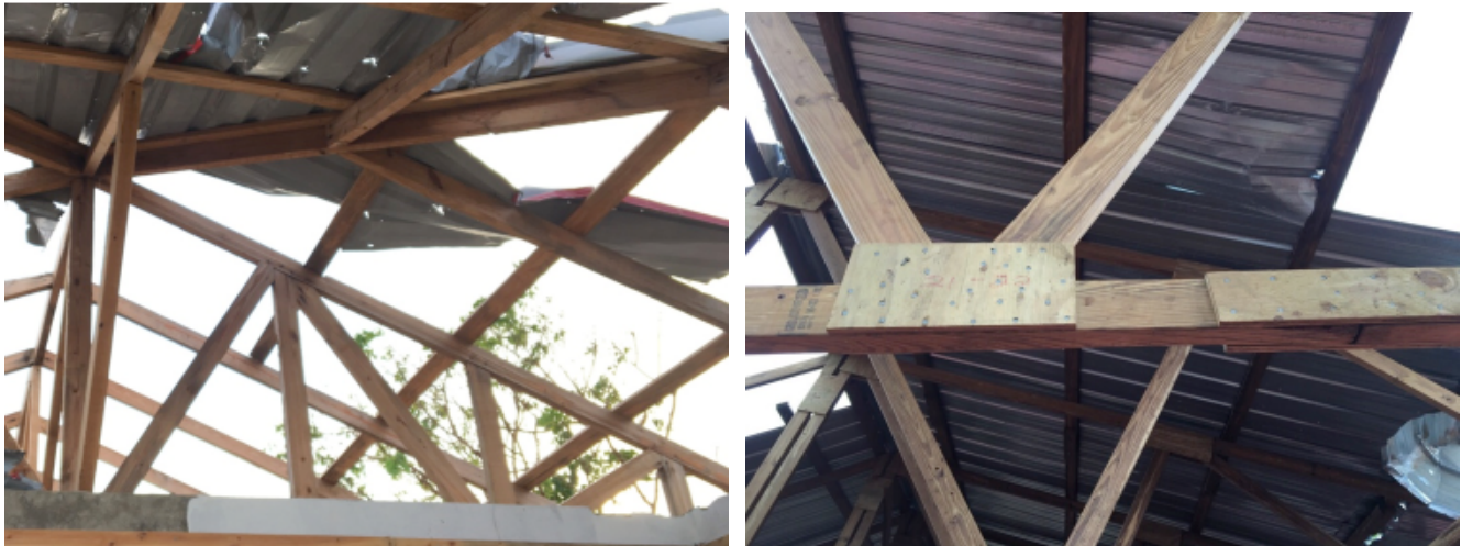
Figure 45 Left: Wood truss with simple nailed connection Right: Wood truss with gusset plate connection
