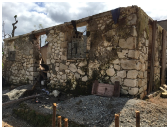
Figure 15 Dry joint stone masonry house in Moron
