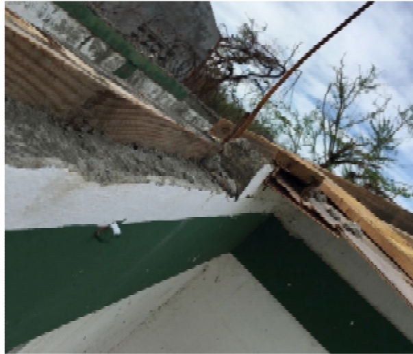
Figure 54 Wood top plate embedded in mortar to connect the roof rafters
