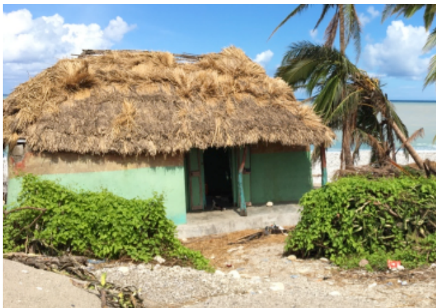
Figure 16 Left: Hipped roof covered of vetiver straw Right: Hipped roof covered of metal sheet
