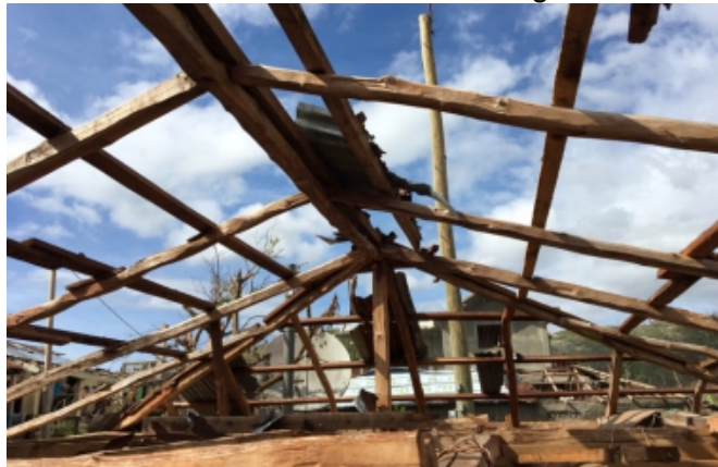
Figure 17 Structure of a hipped roof
