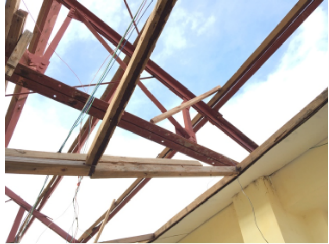
Figure 47 Left: metal sheets blown away right: Roof truss made of angles and metal gusset plates
