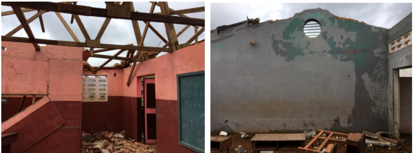
Figure 44 Left: Total collapse of masonry gable. Right: Partial collapse of masonry gable element due to the load from the roof structure.
