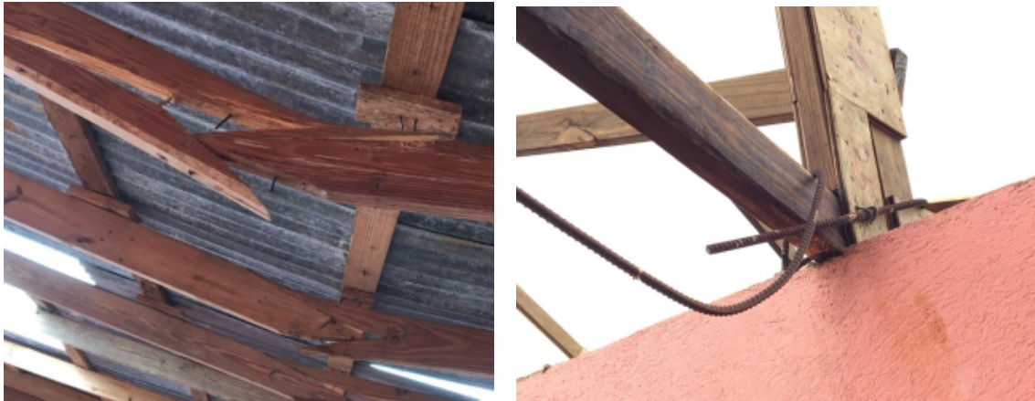
Figure 46 Left: Failure of rafter-to-rafter connection Right: Truss-to-top of the wall connection
