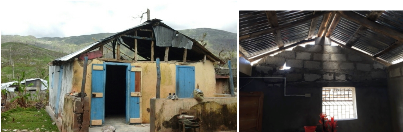
Figure 18 Left: house with a lightweight gable roof Right: Masonry gable wall not confined
