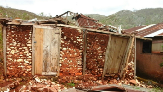
Figure 32 Out-of-plane failure of wall panels
