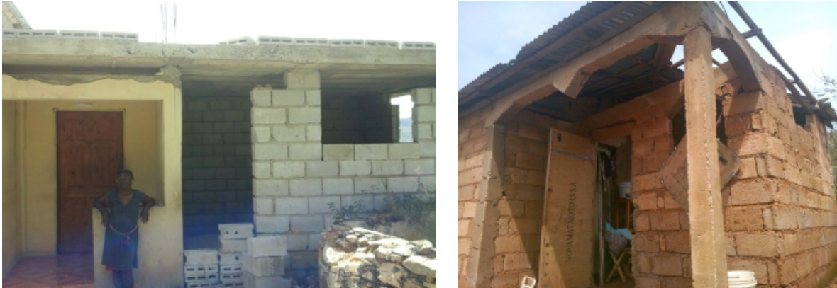
Figure 10 Unreinforced block masonry houses
