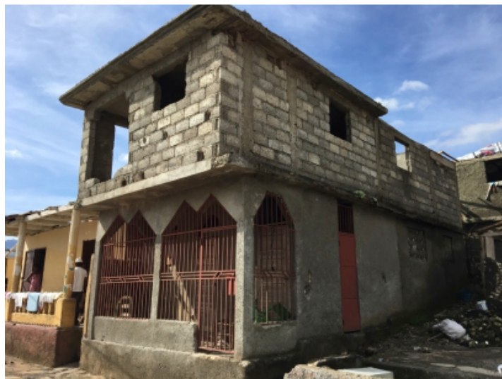
Figure 11 Two-story partially confined block masonry house in Moron
