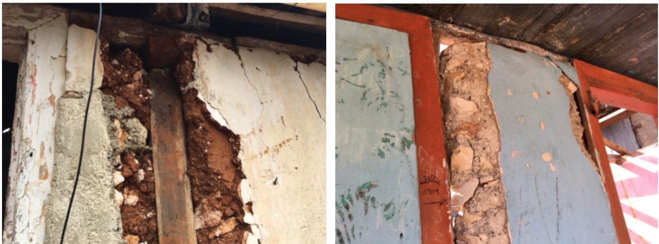
Figure 29 Visible cracks at corner of the masonry
