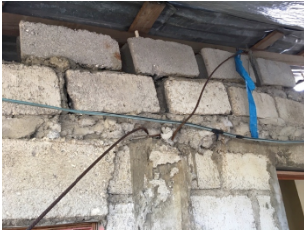
Figure 28 Blocks placed back after the hurricane to replace the roof as the previous ones fell
