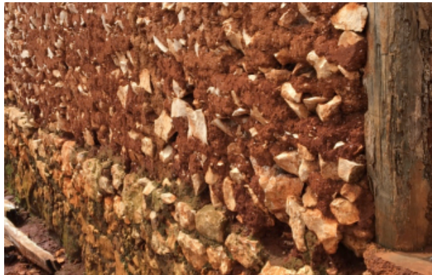
Figure 24 Tuff rocks assembled with mud mortar
