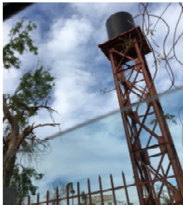
Figure 50 Undamaged steel frame water tower
