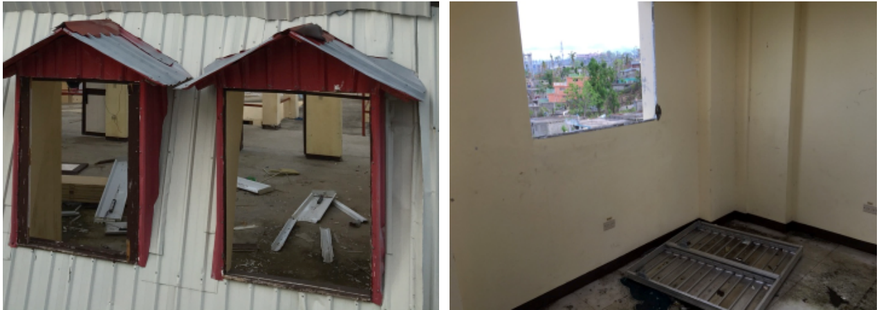
Figure 43 Left: Wood shutters failure Right: Metal louver failure
