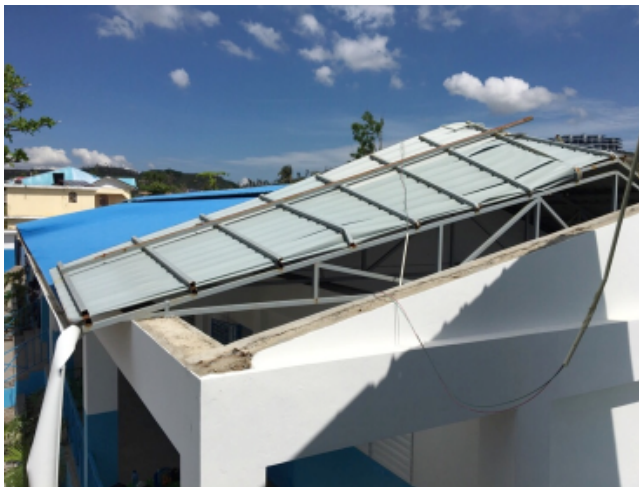
Figure 48 Failure of the welded connection of the masonry gable
