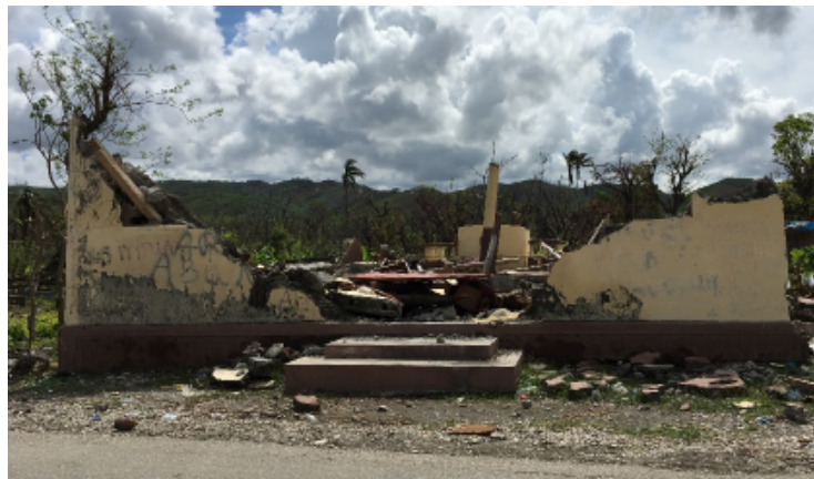
Figure 26 House totally destroyed possibly because of wall failure prior to roof failure
