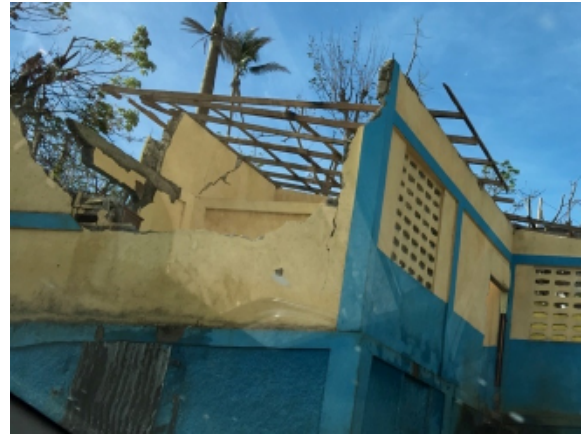
Figure 27 Left: Wall collapse due to lack of tothing and intermediate beam Right: Tall wall collapsed
