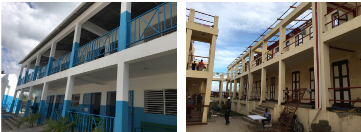
Figure 20 Reinforced concrete frame with block masonry infill schools in Port-Salut (left) and Jérémie (right)
