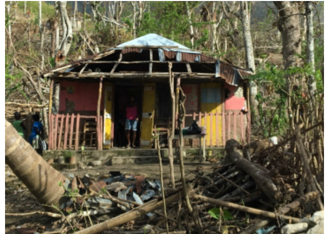
Figure 40 Gallery roof damaged
