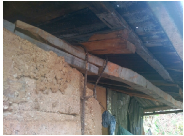
Figure 39 Left: Roof system-to-top plate connection Right: Column-to-top plate connection
