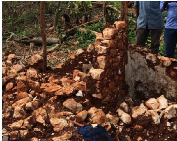
Figure 35 Wall totally collapse due to water infiltration and saturation of mud mortar
