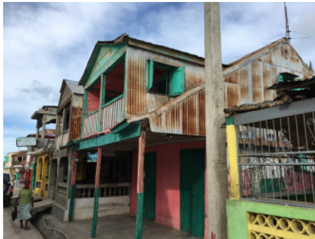
Figure 14 Timber frame vertical expansion with metal sheet panel walls
