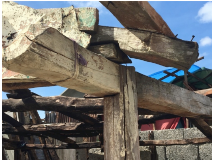
Figure 34 Connection between the ring beam and the top of the wood pole
