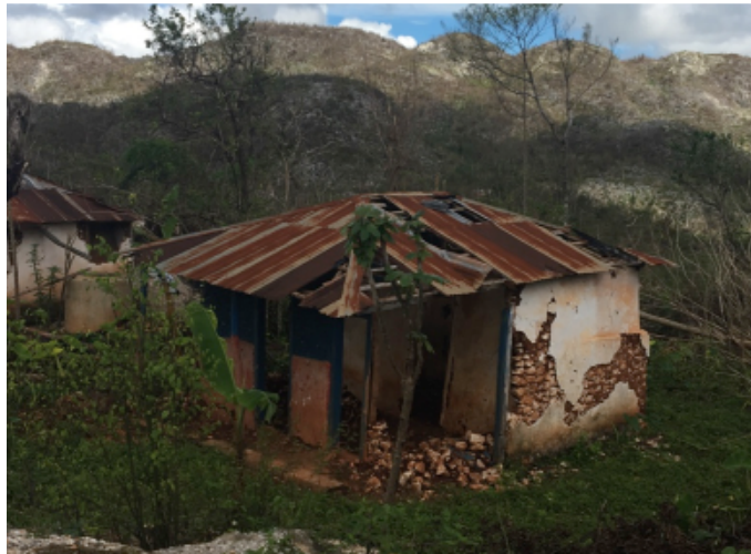
Figure 12 Wood frame with stone masonry infill house
