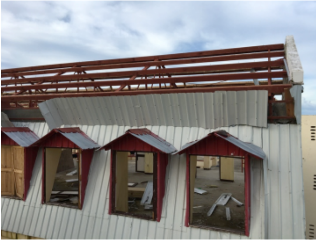
Figure 47 Left: metal sheets blown away right: Roof truss made of angles and metal gusset plates
