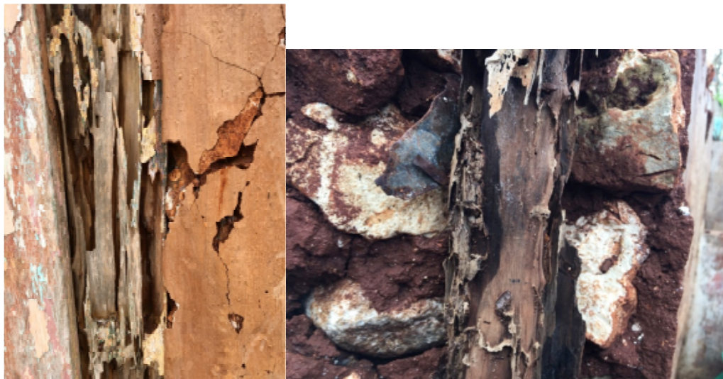
Figure 36 Infested wood poles
