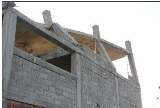
Figure 29. Failure of vertical elements near the column-beam joints, Jama.
