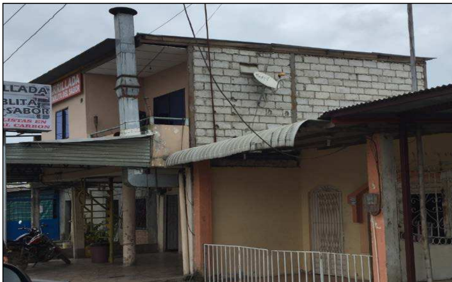
Figure 20. Metal framing with infill concrete blocks wall, outside Guayaquil
