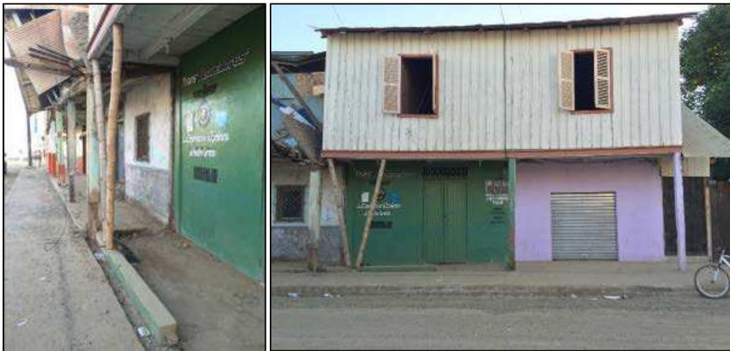
Figure 52. Collapse of timber post, shoring in place, Jama
