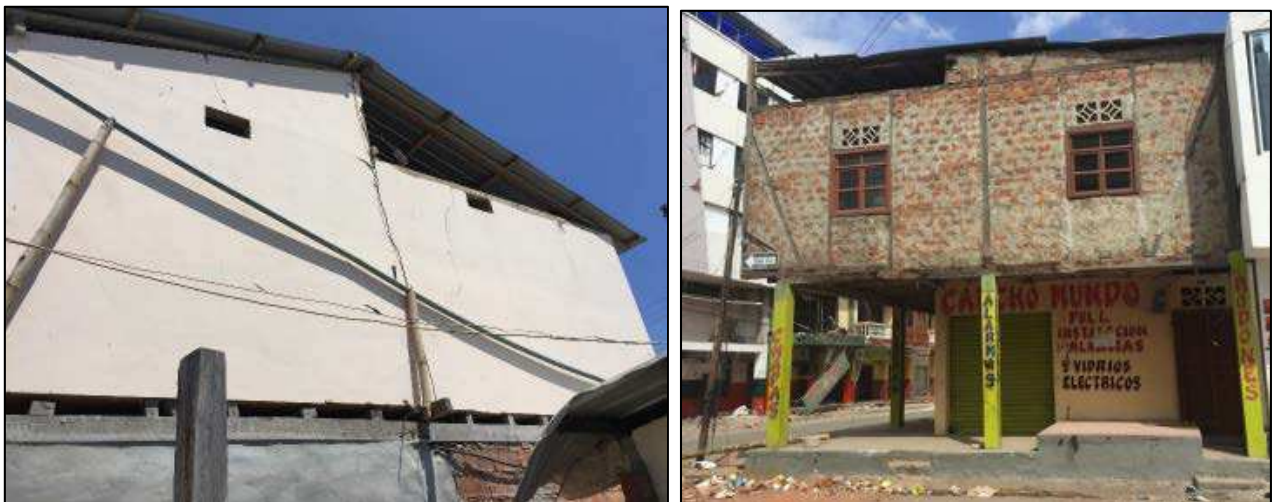
Figure 45. Collapse of infill gable walls, Canoa, left and Manta, right
