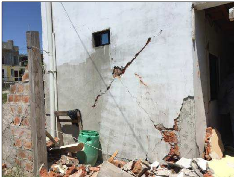
Figure 33. In-plane cracking at end wall, Canoa
