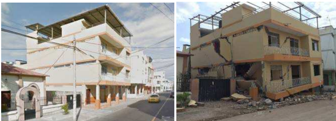
Figure 30. Before (left, source: Google Street View) and after (right) earthquake, Tarqui, Manta.
