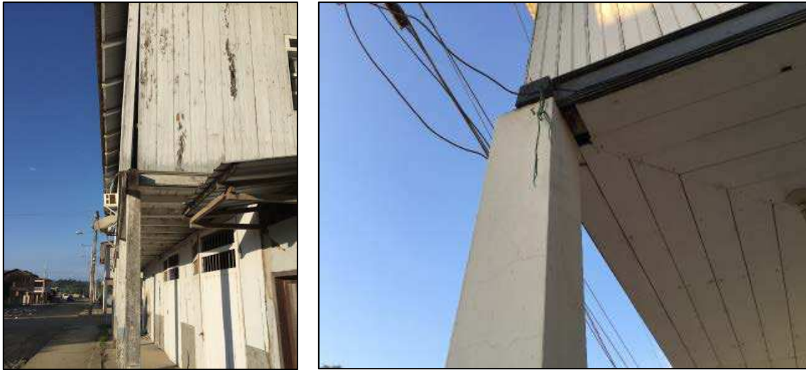
Figure 51. Displacement of posts relative to floor framing, Jama
