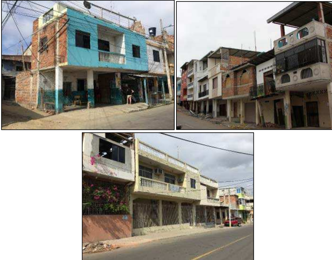
Figure 16. Concrete frames with masonry infill, Manta
