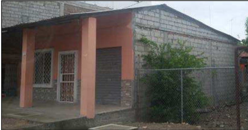
Figure 21. Reinforced Concrete Frames, concrete block masonry and steel elements in the gable wall, outside Guayaquil
