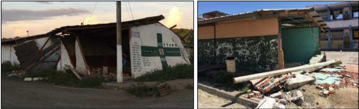
Figure 48. Out-of-plane failure of masonry infill wall in light frame. Jama (left) and Canoa (right)
