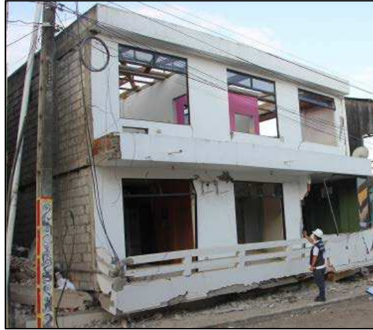
Figure 31. Ground floor collapsed due to soft/weak story failure, Jama.
