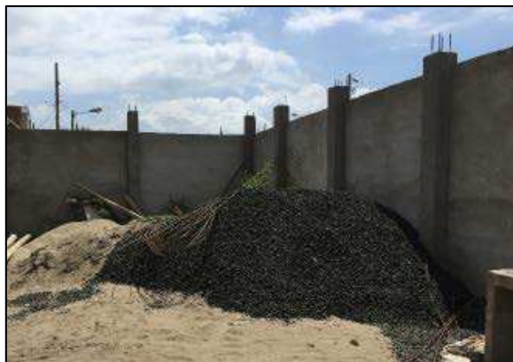
Figure 25. Sand and coarse aggregate stockpiles for informal construction, Crucita
