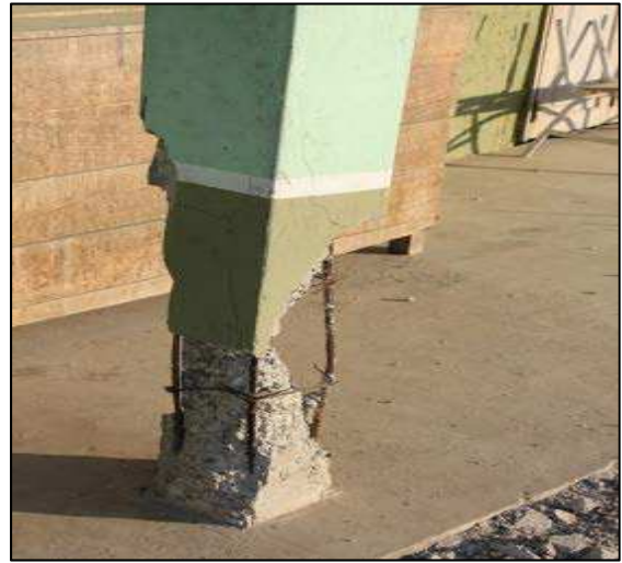
Figure 28. Non-ductile column failure in multi-story building, Manta (left) and single-story building, Jama (right).
