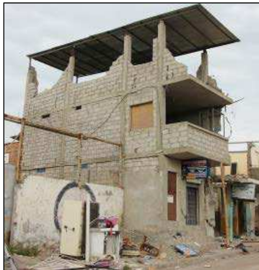
Figure 35. Out-of-plane failure of masonry walls. Lack of ring beam or diaphragm at roof. Manta
