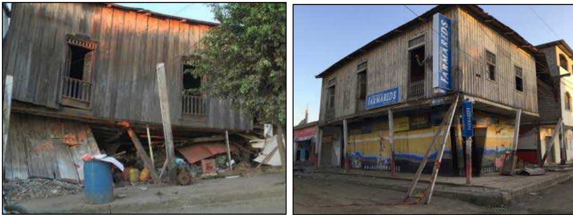
Figure 50. Partial story collapse in timber buildings, Jama
