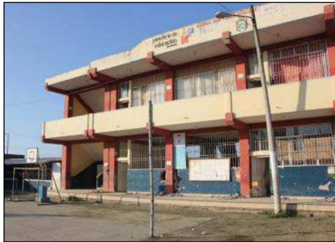
Figure 23. Reinforced concrete frames with infill walls for schools, Jama
