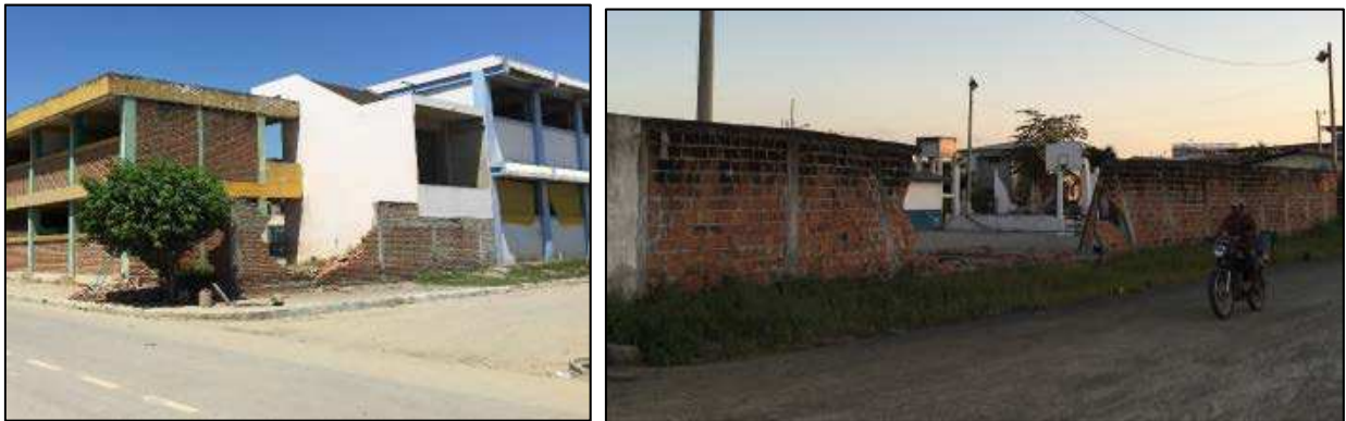
Figure 57. Failure of site walls at schools (Canoa, left and Jama, right)
