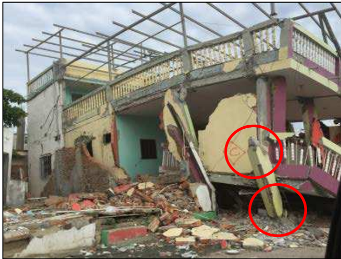
Figure 28. Non-ductile column failure in multi-story building, Manta (left) and single-story building, Jama (right).
