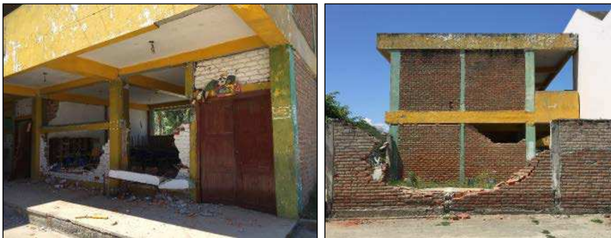
Figure 41. Out-of-plane failure of a classroom walls, Canoa
