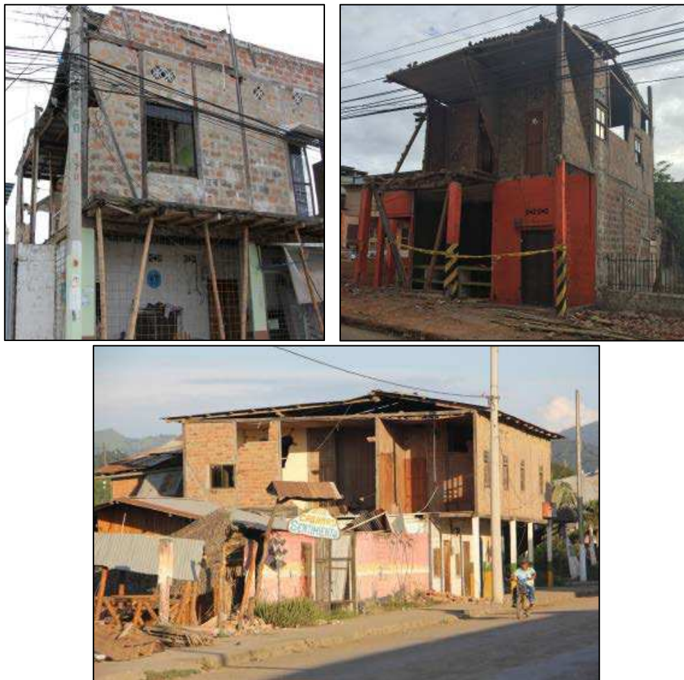
Figure 44. Failure of infill walls. (Manta, top and Jama, bottom)
