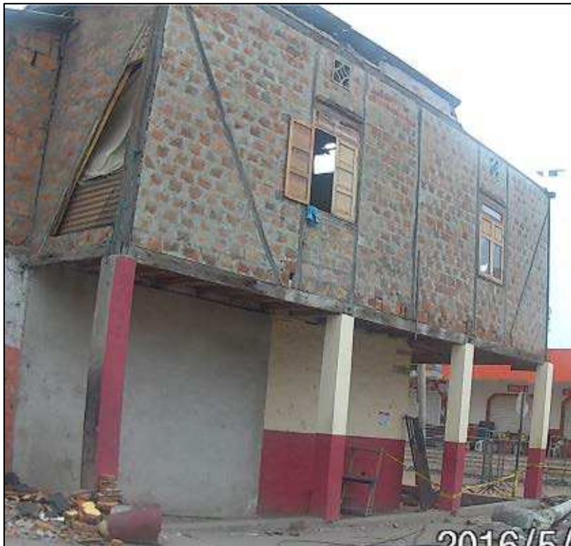
Figure 22. 1 st floor: Concrete frames with infill walls. 2 nd Floor: Timber frames with lateral bracing (In some cases) and infill brick walls. Manta
