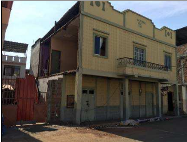
Figure 47. Collapse of wall above decayed floor beam, Los Esteros, Manta
