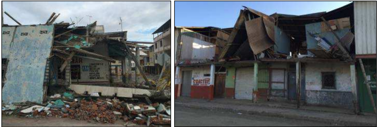
Figure 54. Failure of light-weight walls due to heavier perpendicular walls (Manta, left and Jama, right)
