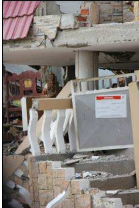
Figure 38. Punching Shear failure / Red Tagged house, Manta.
