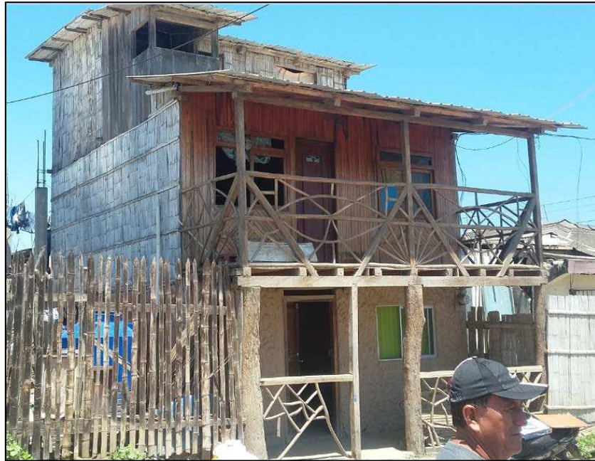
Figure 19. Timber frame and lath walls (Exterior and Interior walls), Canoa
