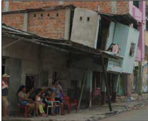
Figure 53. Separation of front façade and overturning, Manta
