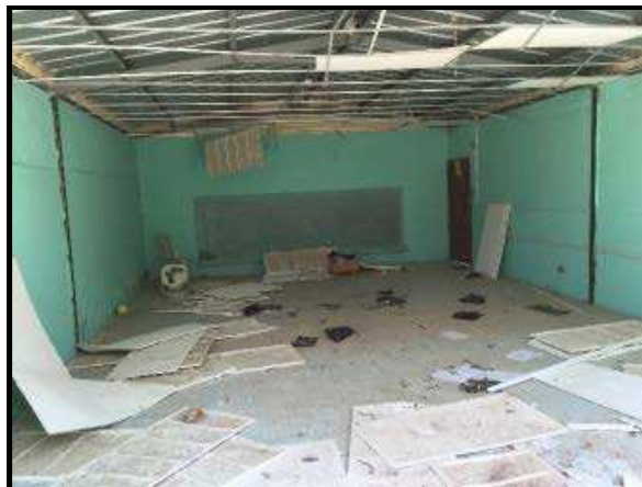
Figure 24. One-story light frame with infill classroom, Canoa
