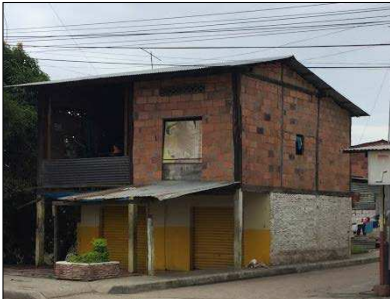
Figure 18. Timber frame with masonry infill walls and lightweight roofs, outside Guayaquil
