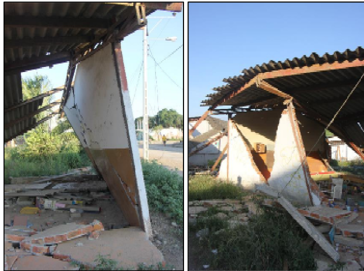
Figure 49. Out-of-plane failure of masonry wall and roof collapse, Jama
