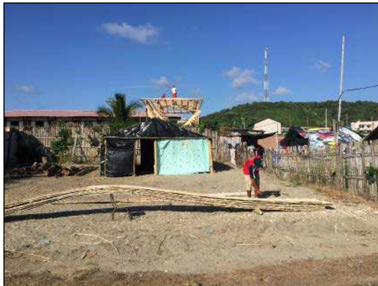
Figure 27. Preparing bamboo lath, Canoa
