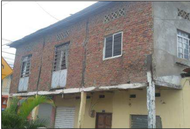
Figure 17. Timber frame with masonry infill walls and lightweight roofs.
