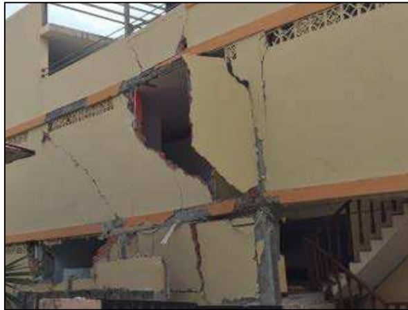
Figure 34. Out-of-plane failure of masonry walls. Perforated block/vent at wall panel connection to slab. Manta
