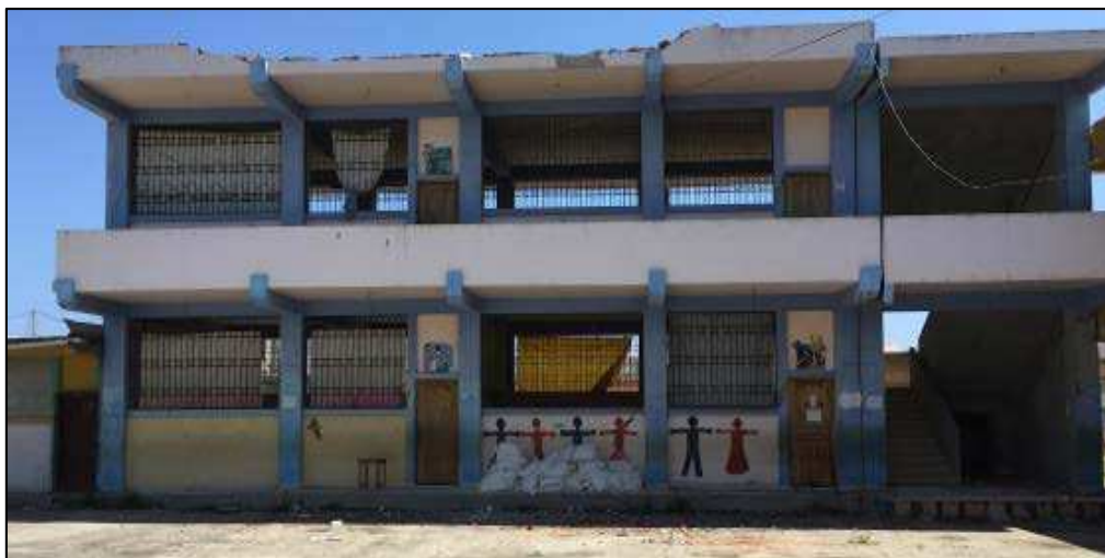
Figure 43. Parapet collapse at a school building, Canoa
