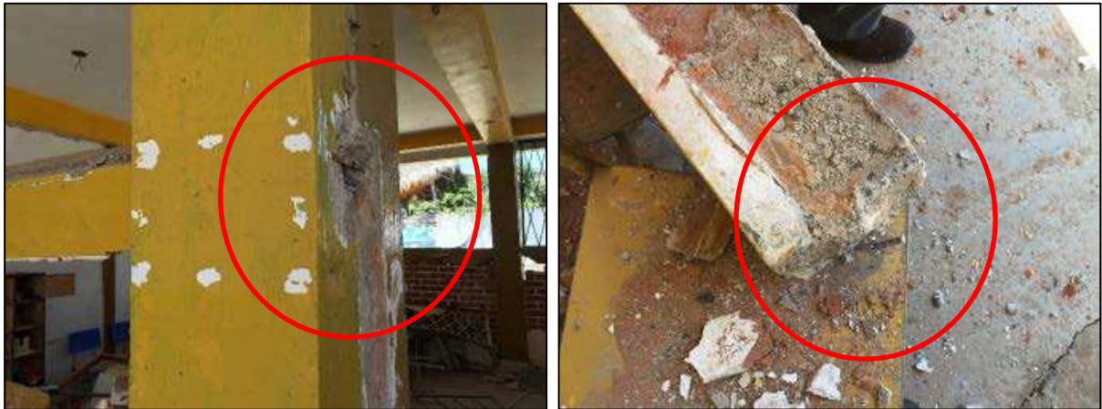
Figure 42. Connection failure of wall panel bracing element, Canoa
