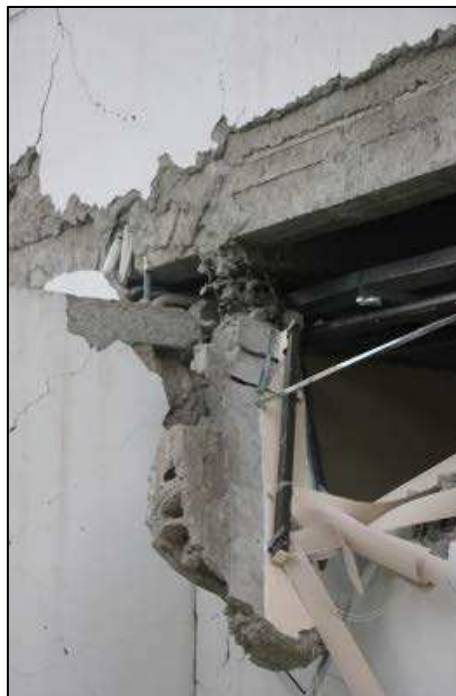
Figure 37. Short Column failure. Outside Canoa
