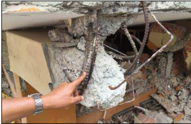
Figure 26. Typical reinforcing exposed in damaged column, Tarqui, Manta
