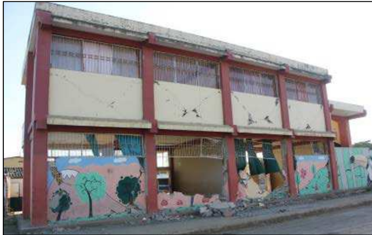
Figure 40. Cracking and failure of non-structural elements at a school, Jama
