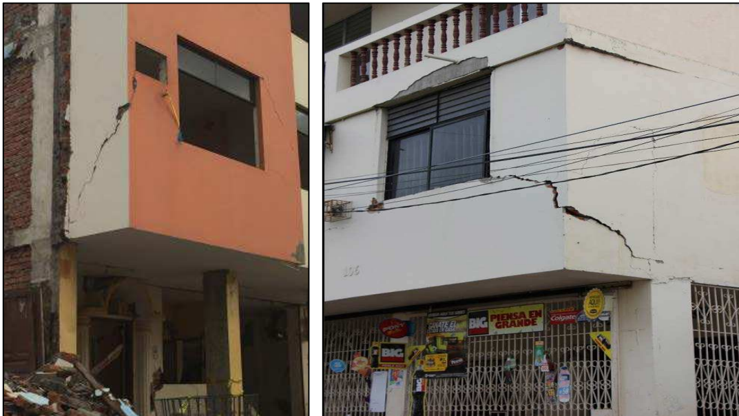
Figure 36. Failure at the overhangs, Manta
