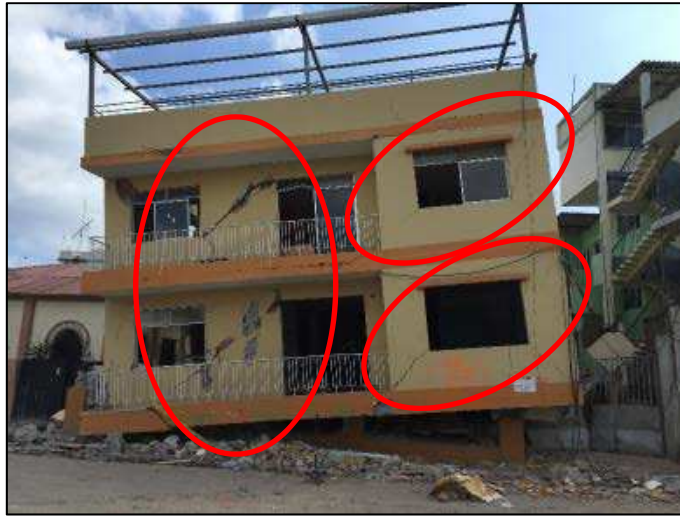
Figure 32. In-plane masonry infill wall cracking, Tarqui, Manta
