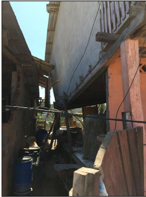
Figure 46. Wood frame connections failure, loss of support, Canoa
