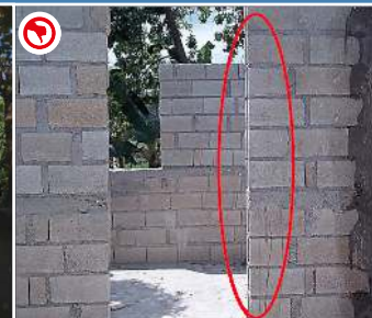
Use a column at the edge of door openings.
