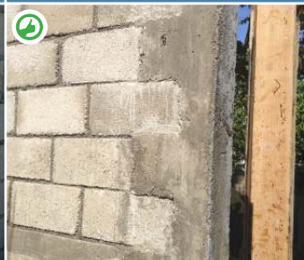
Use a column at the edge of door openings.
