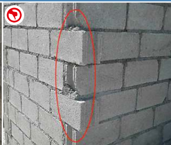
Use columns at every wall intersection and corner.
