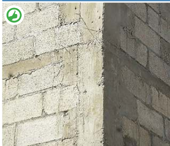
Use columns at every wall intersection and corner.
