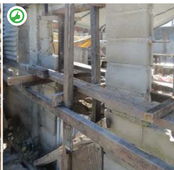
Coconut lumber can be used for scaffold and shoring
