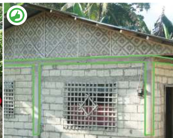
Use a ring beam on top of walls.
