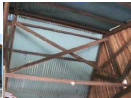
A gable roof can also be built to be typhoon resistant, however this configuration requires diagonal bracing for it to be stable
