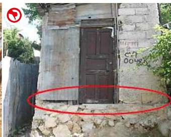
Use a plinth beam at the base of walls.
