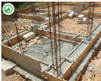
Use a plinth beam at the base of walls.
