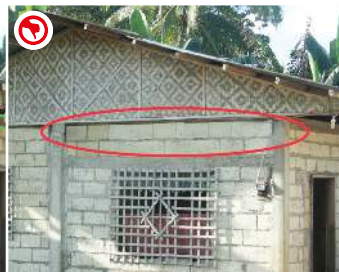
Use a ring beam on top of walls.
