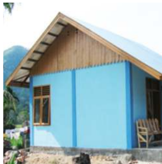
A gable roof can also be built to be typhoon resistant, however this configuration requires diagonal bracing for it to be stable
