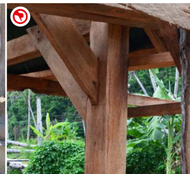
Do not use coconut lumber for structural members - it may not be strong enough and deteriorates too fast
