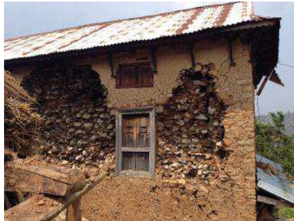
Figure 76. Delaminated wall failure, Mahankal Chaur VDC
