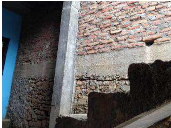
Figure 105. School with concrete frame and infill with brick and stone, with a beam poured on top, Chalal Ganeshthan VDC
