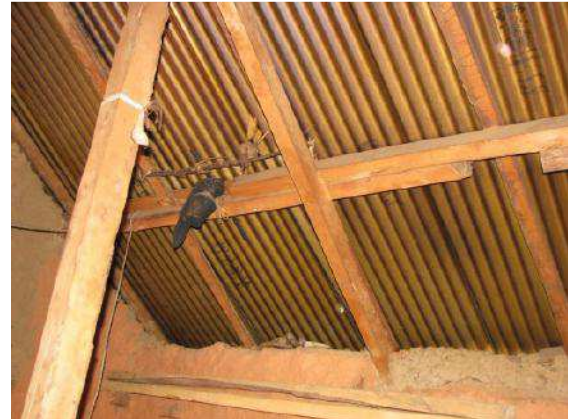
Figure 40. CGI over sloped timber roof framing, Thula Gaun.
