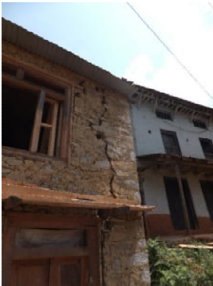
Figure 77. Cracks through holes in walls, Dhungharka VDC
