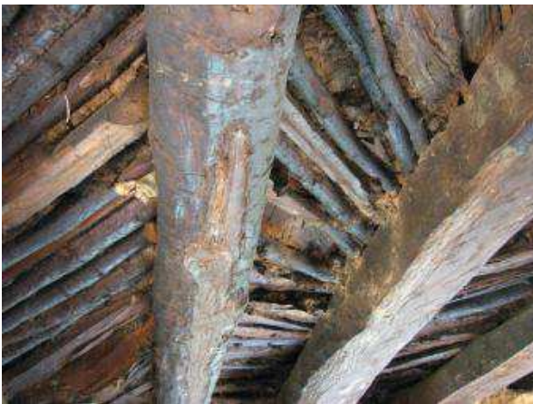
Figure 35. Herringbone subfloor layout, Thula Gaun.
