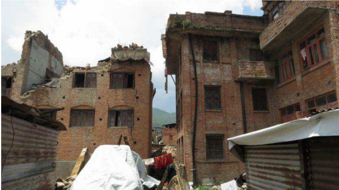
Figure 48. Sankhu - Both buildings are 3-4 stories, with wood floors and fired brick walls. The building on the left utilized mud mortar and sustained significant damage, while on the right the building used cement mortar and had no observable damages.
