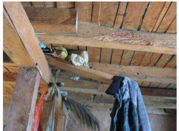
Figure 36. Straight sheathed subfloor, Thula Gaun.
