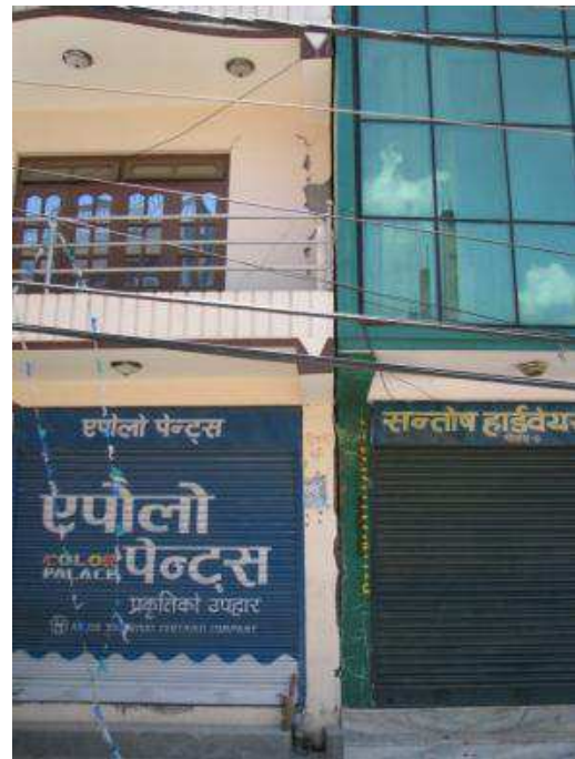
Figure 57. Pounding damage, Chautara.
