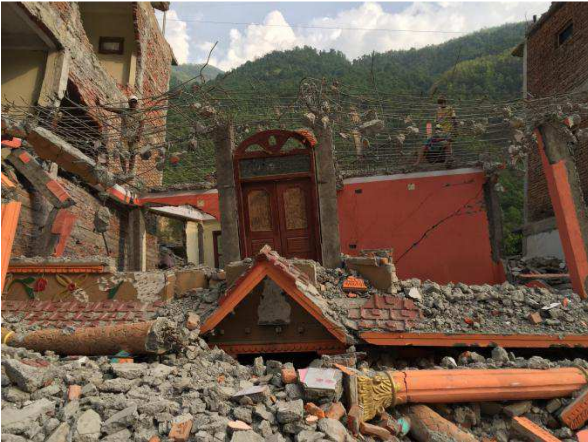
Figure 60. Demolition of collapsed building. Note damage to adjacent building caused by building collapse, Khadichaur.
