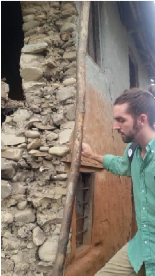
Figure 109. Partially collapsed mud in stone house
