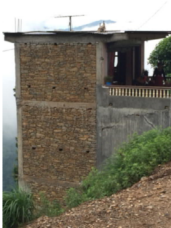
Figure 87. Reinforced concrete frame with stone and mud infill encountered in the rural area of Nuwakot.
