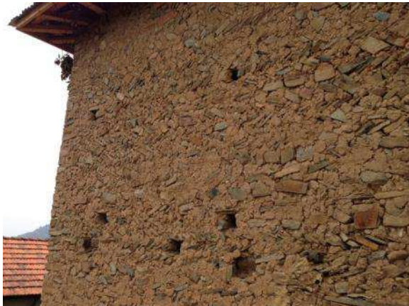
Figure 31. Stone wall construction, Chahal Ganeshtan, Kavrepalanchok
