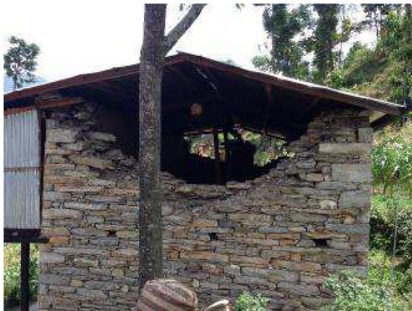
Figure 73. Out of plane wall failure, Ramche VDC
