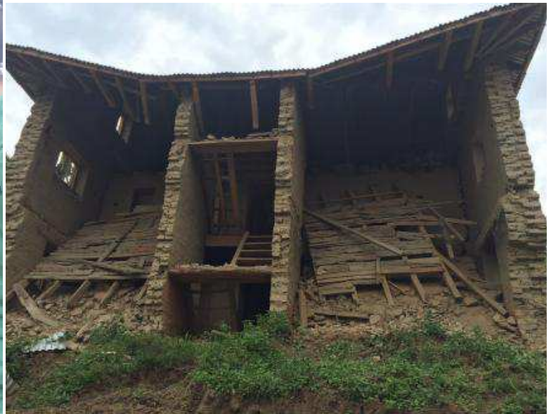
Figure 110. Partially collapsed adobe house in Devi Chaur
