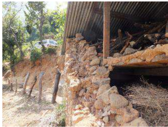
Figure 74. Out of plane wall failure, Dhungharka VDC
