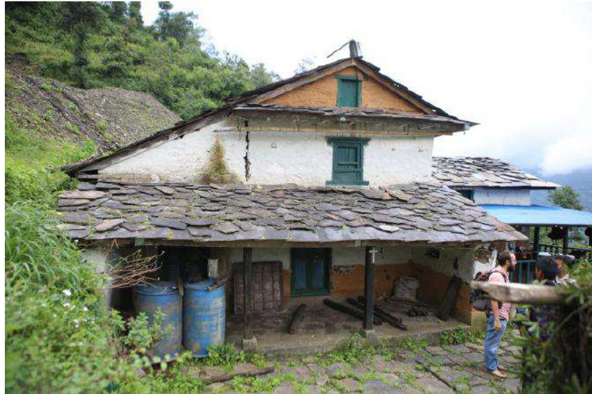
Figure 89. Typical house in Ragani constructed from stone and mud, damaged
