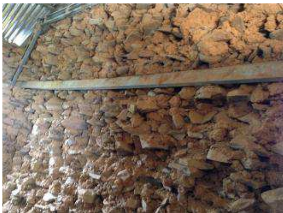
Figure 101. Delaminated stone masonry wall in school, Chalal Ganeshthan VDC
