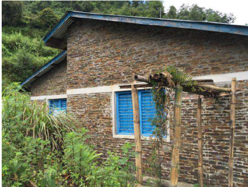
Figure 91. Medical center in Ragani built with stone, cement mortar, and a concrete band at the lintel level.
