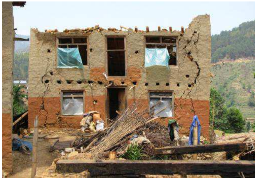
Figure 69. Severely damaged stone masonry home with randomly shaped rocks, Thula Gaun.
