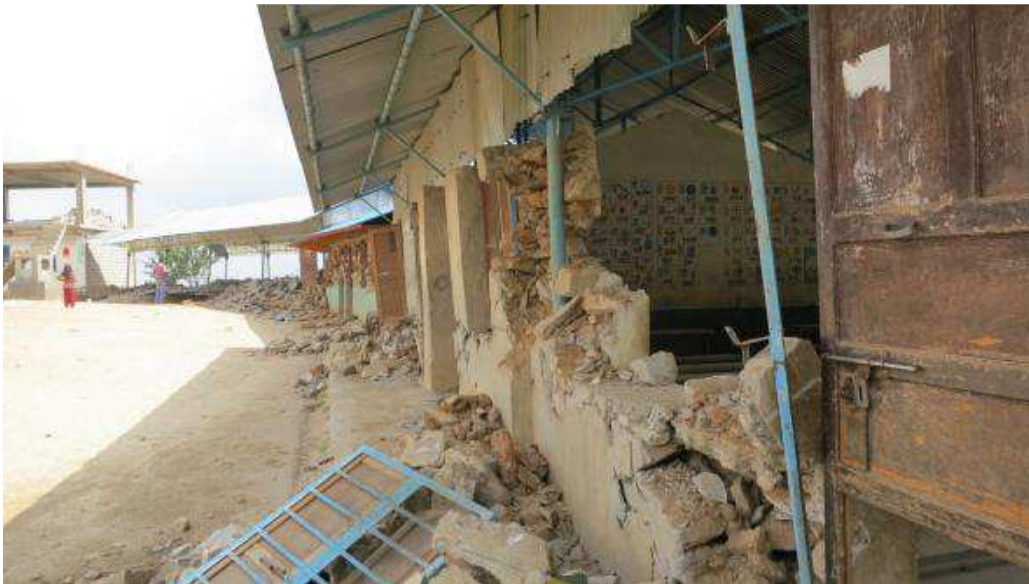
Figure 98. Damaged single-story structures at school, Ichok.
