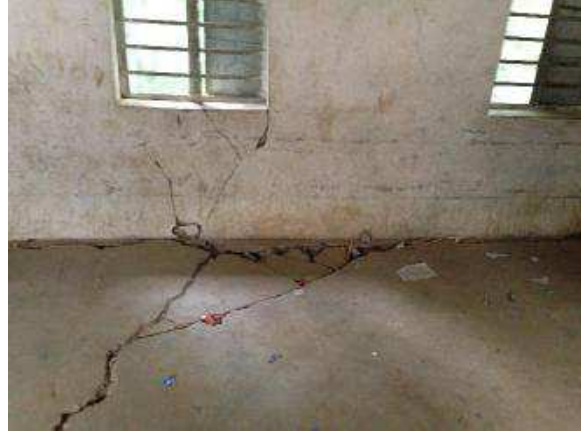
Figure 80. Undermined foundation slab in school, Chyasingkharka VDC
