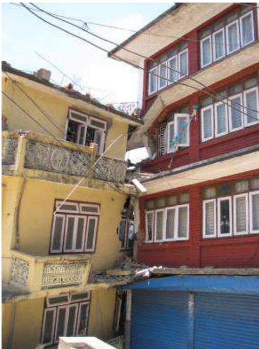
Figure 56. Damage due to adjacent building collapse, Chautara.
