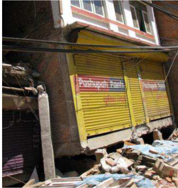
Figure 51. Foundation/lower level failure on hillside, Chautara (See Figures 52 & 53 for column failure details).
