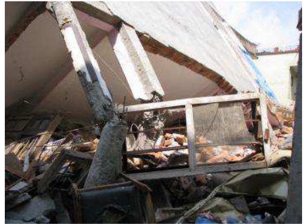
Figure 42. First story column failure, Balkhu.
