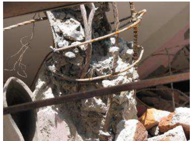
Figure 43. Close up of Figure 35 column failure, Balkhu.
