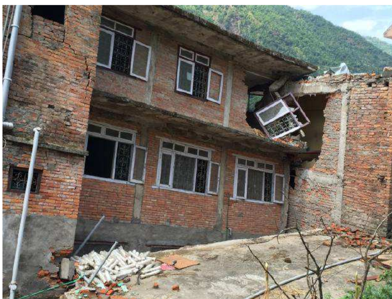
Figure 59. Damage due to collapse of adjacent building, Lamosanghu.
