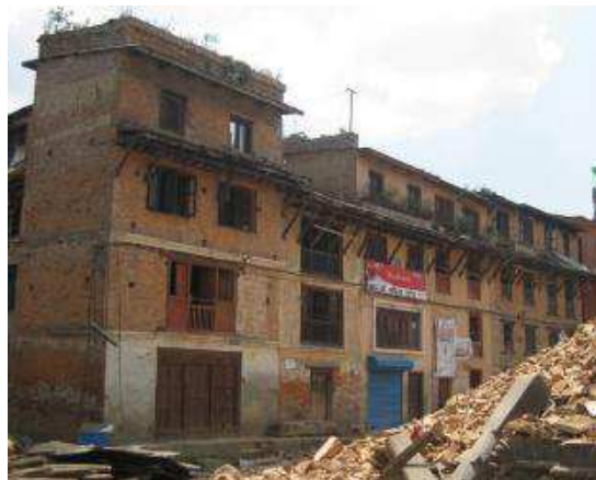
Figure 15. Urban area unconfined, unreinforced masonry buildings,
