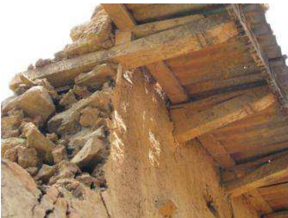
Figure 35. Herringbone subfloor layout, Thula Gaun.
