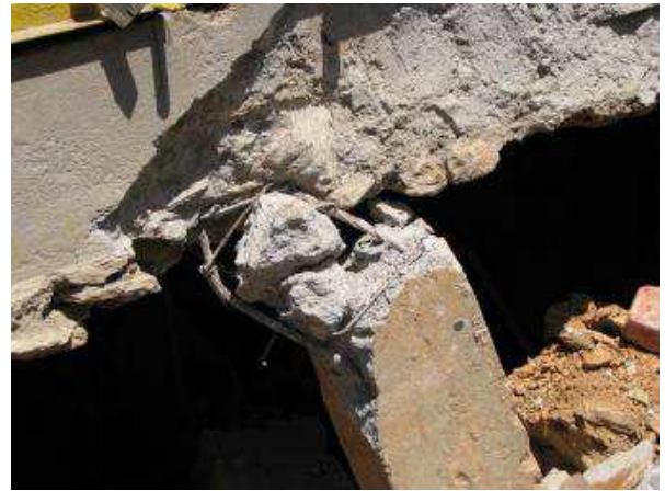
Figure 53. Foundation column failure, Chautara.
