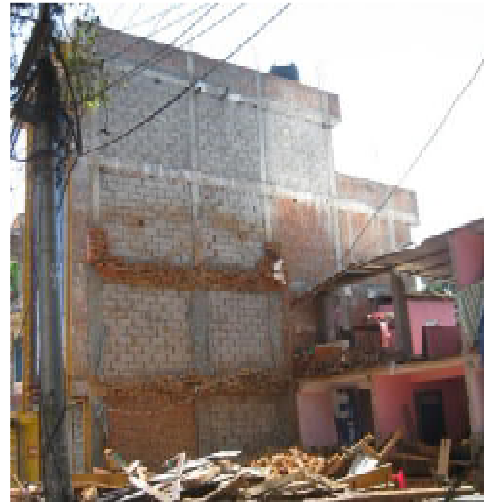
Figure 14. Concrete block infill, Chautara.
