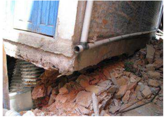
Figure 55. Foundation failure, Chautara.
