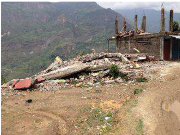
Figure 81. Collapsed concrete frame house, Maneshwor VDC
