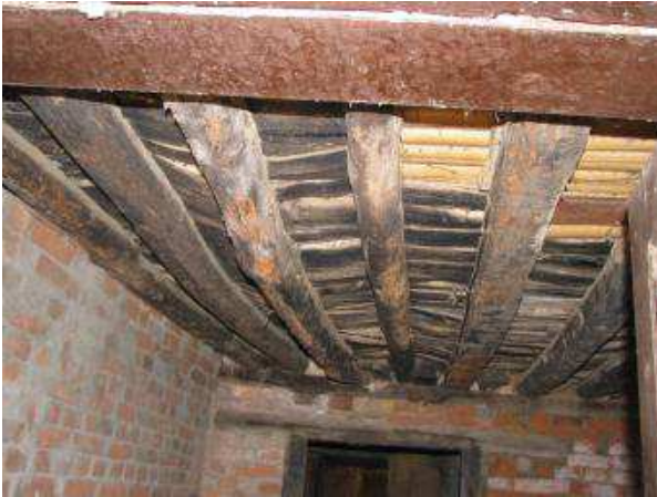
Figure 33. Example of subfloor framing, Bungamati.
