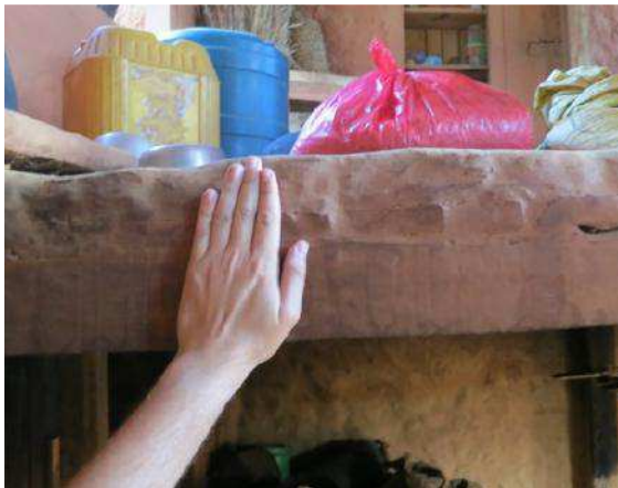
Figure 39. Mud floor over straight sheathed subfloor.
