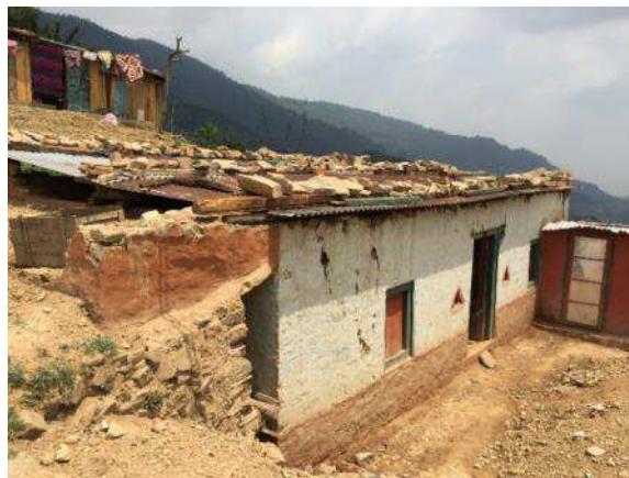
Figure 66. One of the houses in Chalal Ganeshthan Ward 9 where the upper floors were demolished and the ground floor level covered with CGI sheets.
