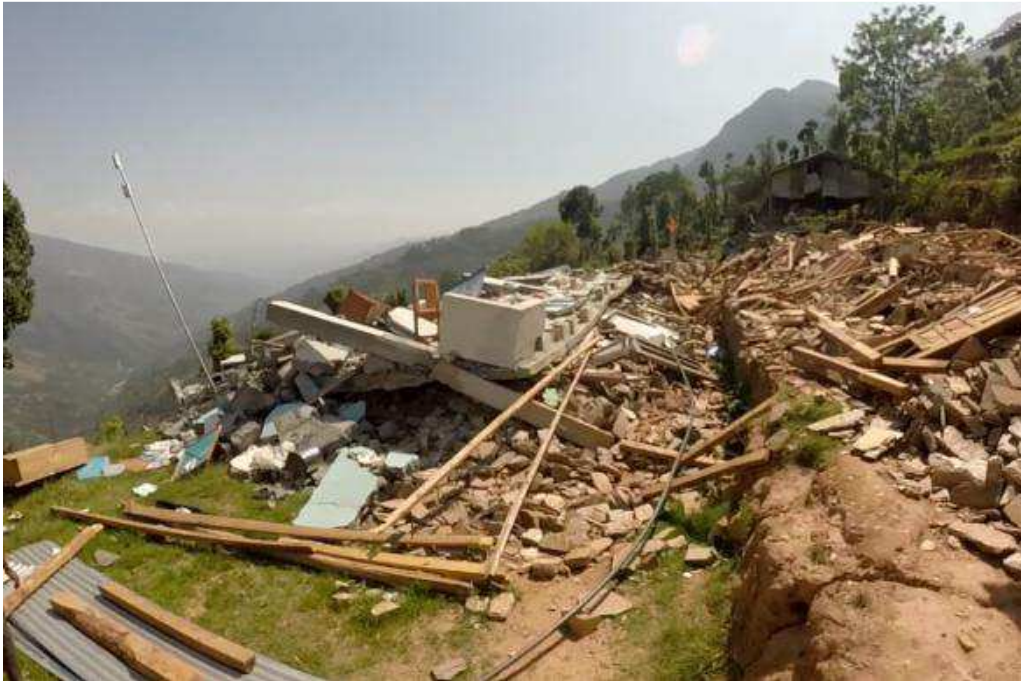
Figure 111. Completely collapsed two-story concrete frame with infill school, Baruwa
