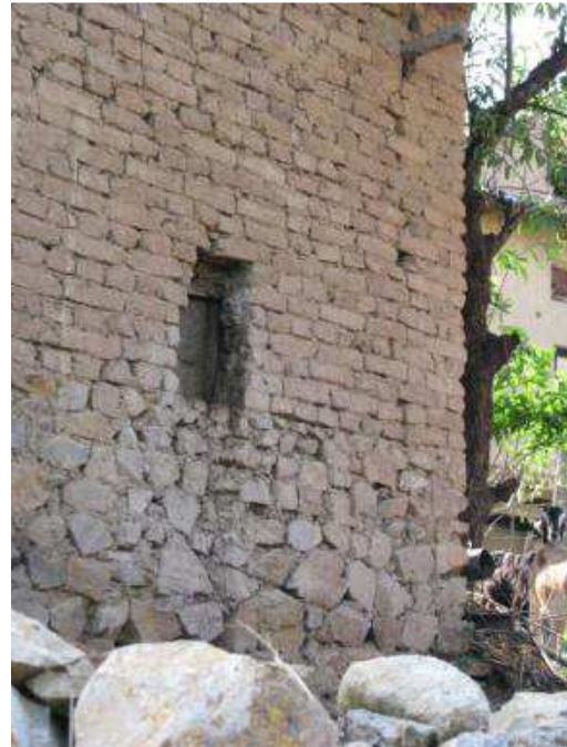
Figure 17. Brick above stone masonry, Zero Kilo.
