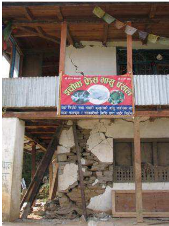
Figure 71. Large cut stones in damaged stone masonry, with plaster over stonework, Ichok.
