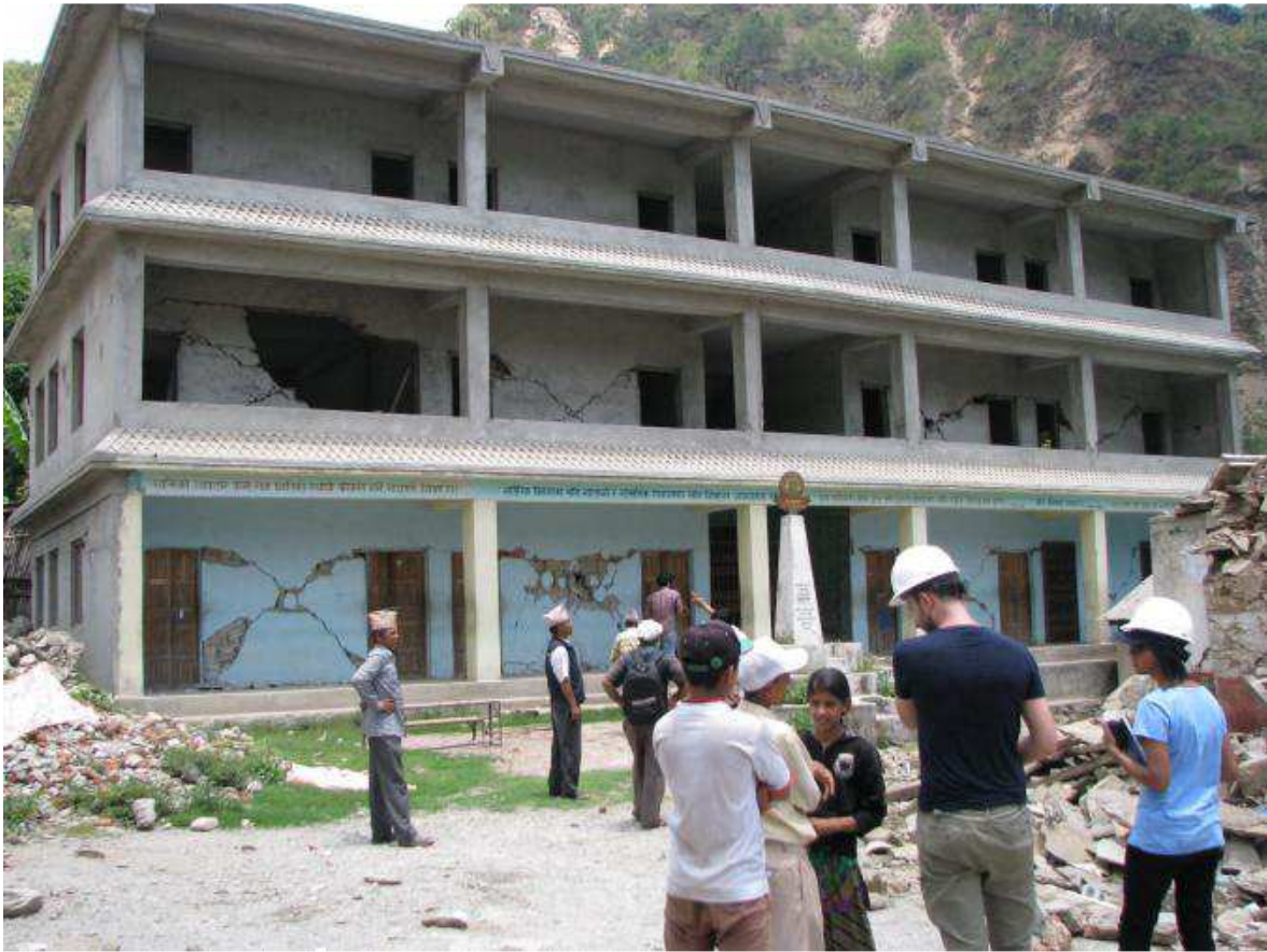
Figure 94. 3-story concrete frame Shree Saraswati School structure with shear cracking at infill walls, Mahankal.
