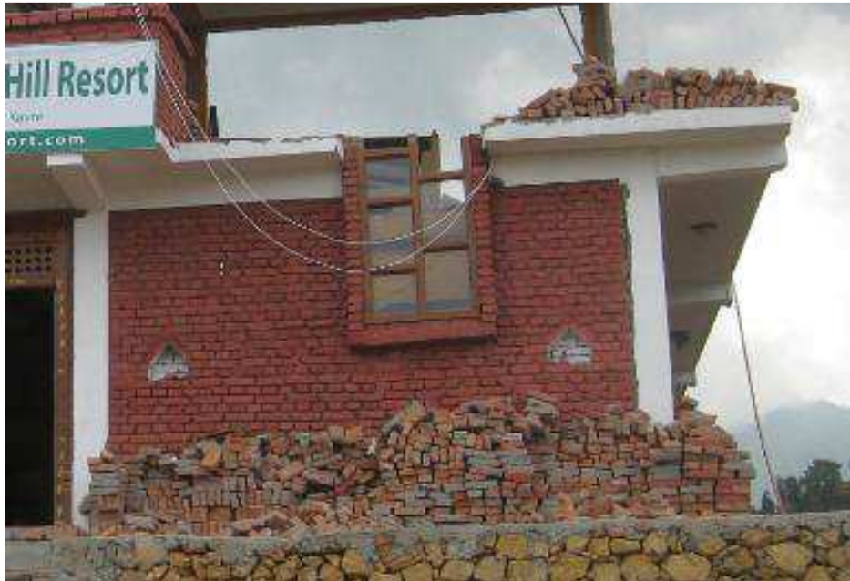
Figure 113. Construction of non-continuous, non-code complying beam at stairway of hotel structure in rural area, Thula Gaun.
