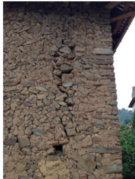
Figure 78. Cracks through holes in walls, Chalal Ganeshthan VDC
