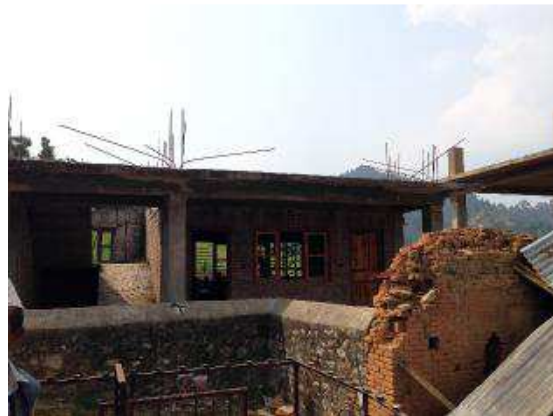
Figure 106. Concrete frame school building under construction in Mahankal Chaur
