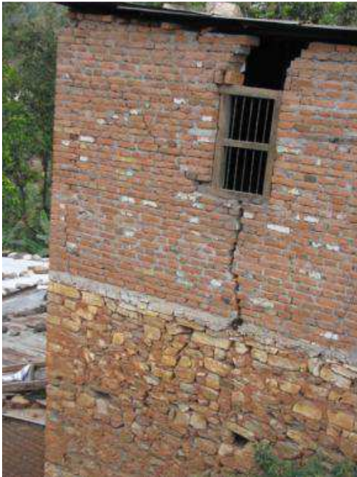
Figure 16. Brick above stone masonry, Balthali VDC.
