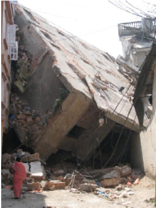
Figure 41. Soft story failure, Kuleswor.
