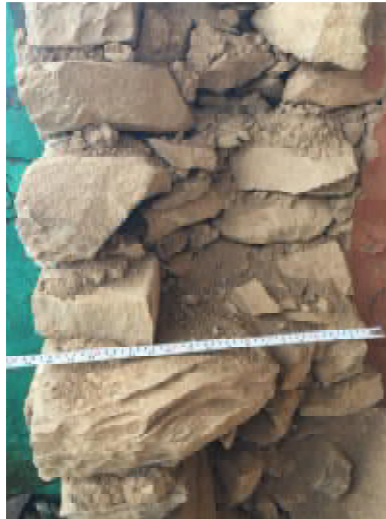
Figure 88. Wall section of a collapsed stone and mud structure, Kaule.
