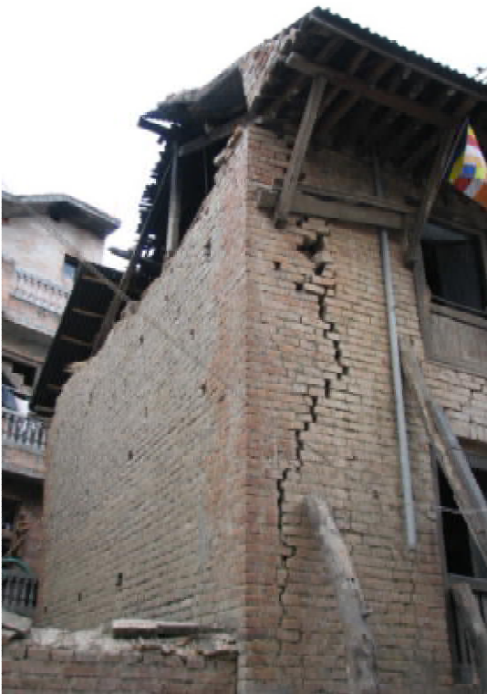
Figure 44. Gable wall failure & corner separation, Khokana.
