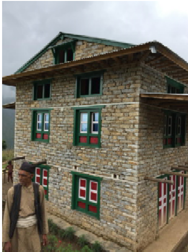
Figure 90. Exceptional stone work for stone and mud mortar building found in Chaulakharka, minimal damage
