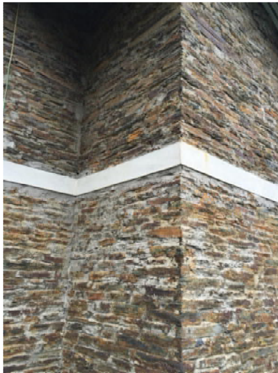
Figure 92. Stone with cement mortar and concrete band at medical center in Ragani
