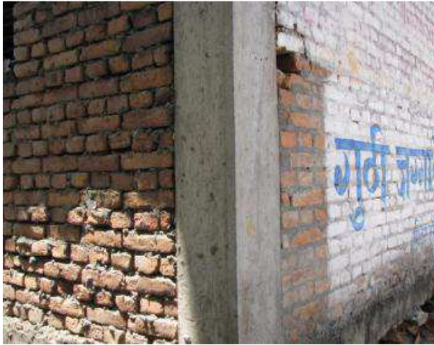
Figure 13. Note mortar finishing on exposed side wall versus mortar finish on “out of sight” back wall, Chautara.
