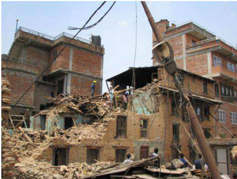
Figure 47. Unconfined masonry collapse. Note undamaged infilled frame in background, Khokana.
