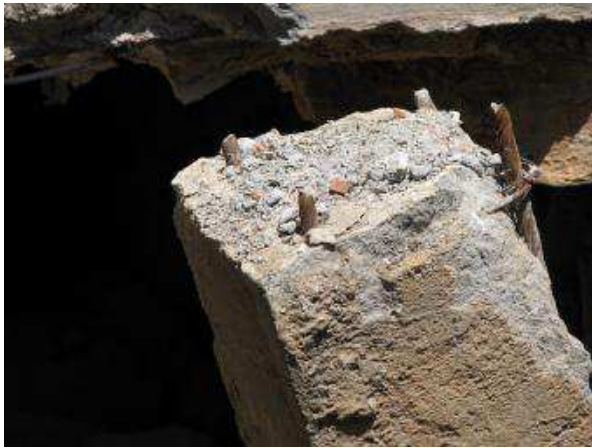
Figure 52. Foundation column failure, Chautara.
