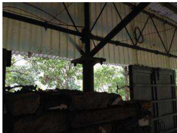
Figure 102. School with steel framed roof and stone masonry walls, Ramche VDC
