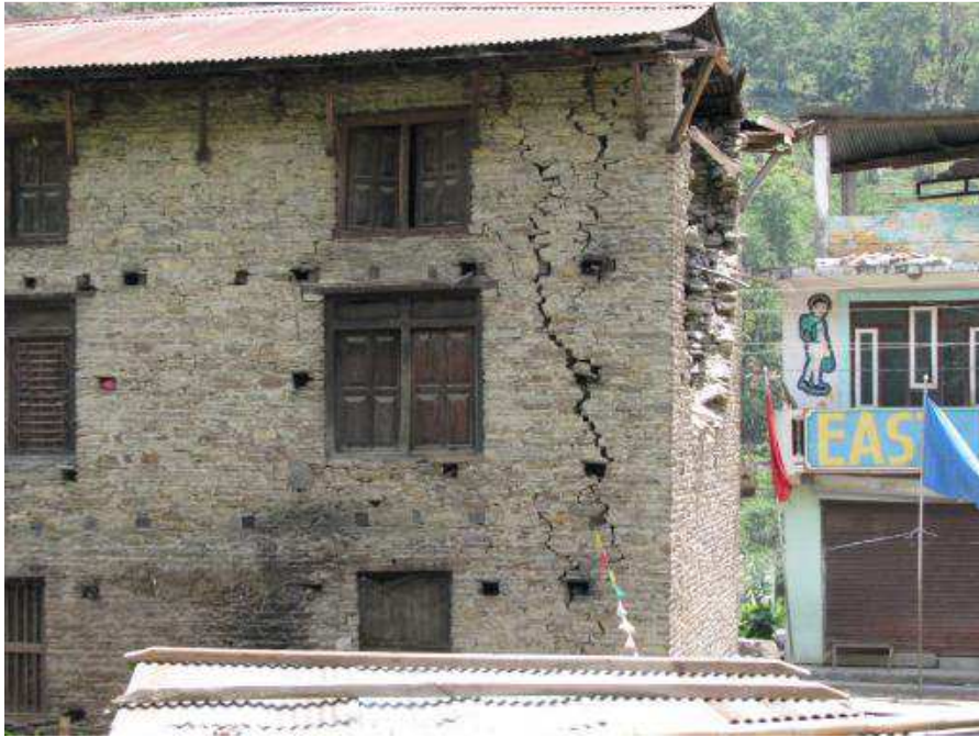
Figure 70. Damaged stone masonry with small cut stones, Mahankal, Sindhupalchok.
