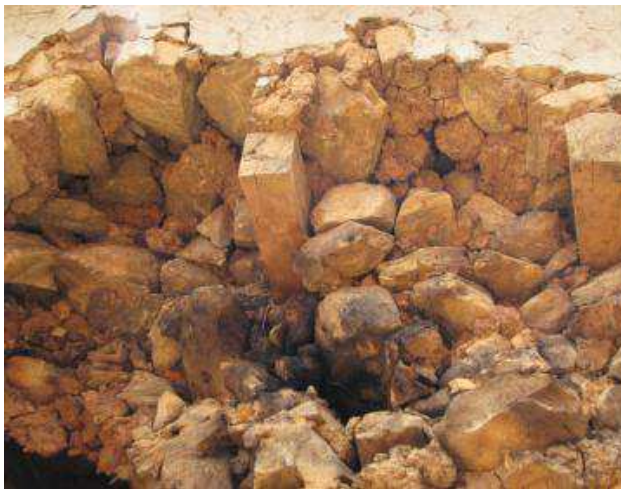
Figure 20. Random shaped stone masonry, Thula Gaun.
