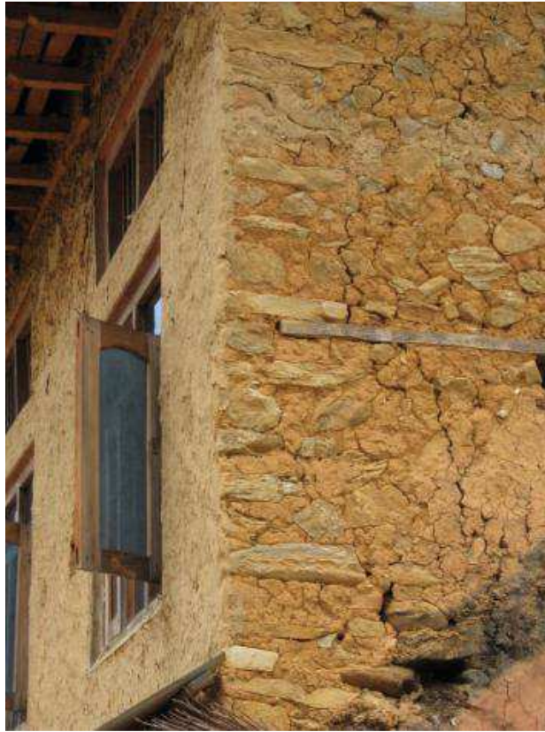
Figure 28. Example of flat cut stone with random stone shapes, Thula Gaun.
