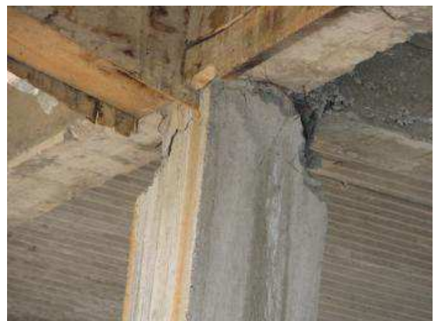
Figure 100. Beam-column connection damage, Ichok.
