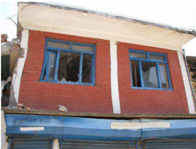
Figure 58. Damage due to pounding and collapse of adjacent building, Chautara.
