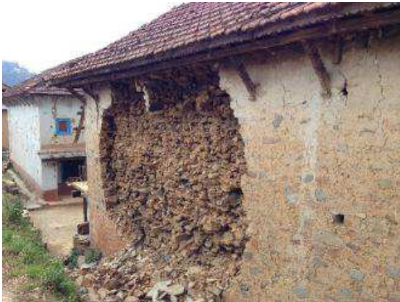
Figure 75. Delaminated wall failure, Chalal Ganeshthan VDC
