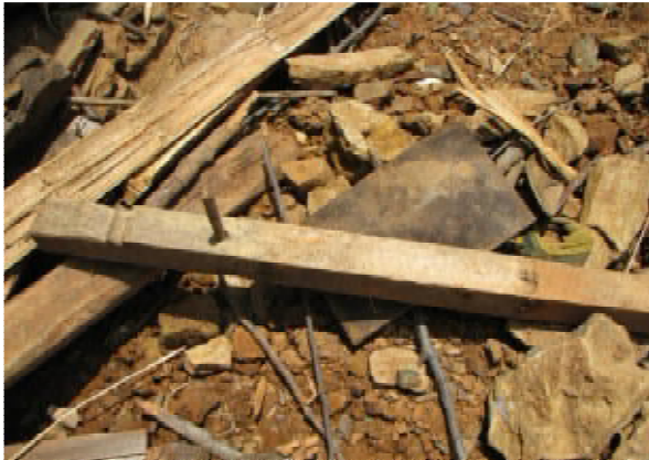
Figure 38. Pegged rafter in rubble pile, Thula Gaun.
