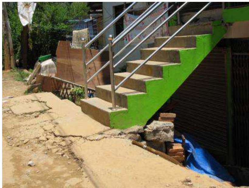
Figure 50. Evidence of foundation shifting at front of building (bottom of stair), Chautara.
