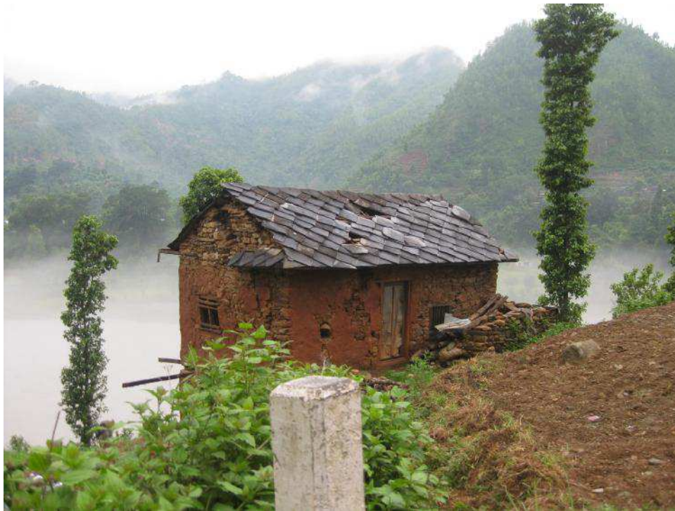
Figure 85. Example of a typical damaged stone and mud house with slate tile roof, Lachyang.
