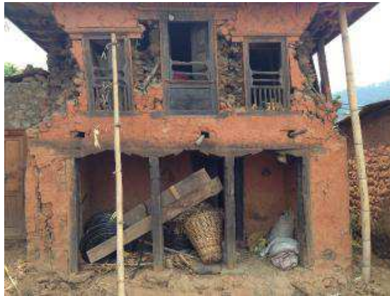
Figure 72. House with major damage at the corners, Mahankal Chaur VDC
