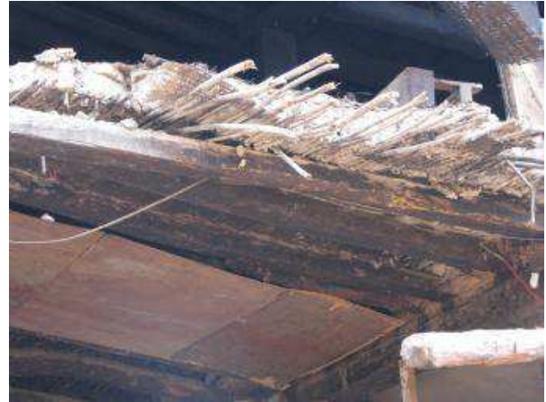
Figure 34. Example of subfloor framing, Bungamati.
