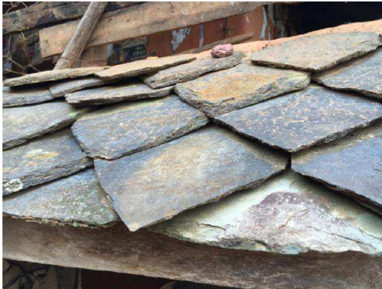
Figure 86. Example of slate roofing that has been cut into smaller tiles, Lachyang.
