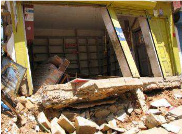
Figure 54. Foundation failure, Chautara.
