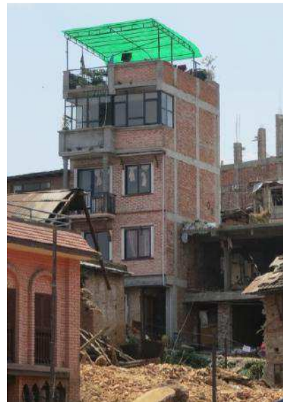
Figure 12. Reinforced concrete frames with masonry infill.
