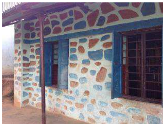
Figure 103. School in Dhungharkha with a horizontal band over the windows and doors
