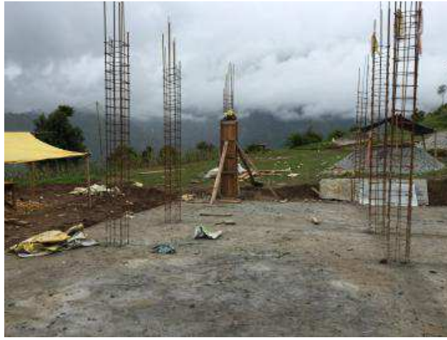
Figure 93. Reinforced concrete frame structure being constructed in Chaulakharka
