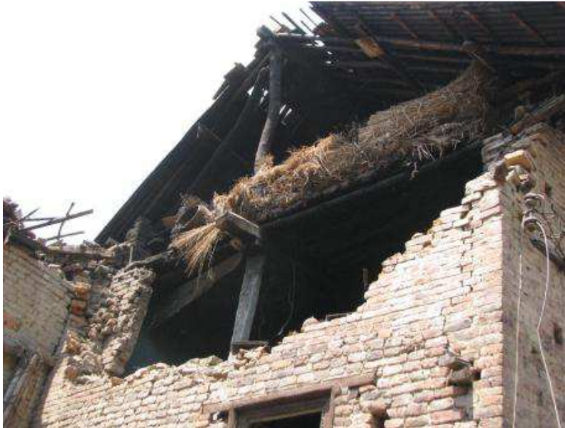
Figure 46. Collapsed end wall at gable, Bungamati.
