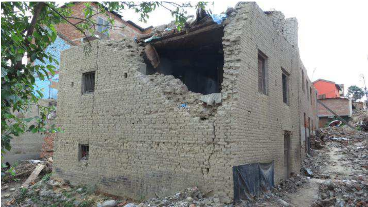
Figure 24 Damaged unfired brick and mud house in Sankhu
