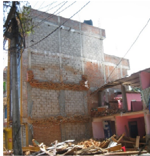
Figure 14. Concrete block infill, Chautara.
