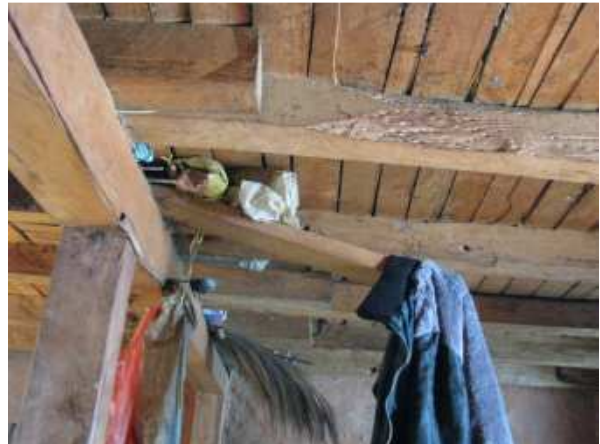
Figure 29. Straight sheathed subfloor, Thula Gaun.
