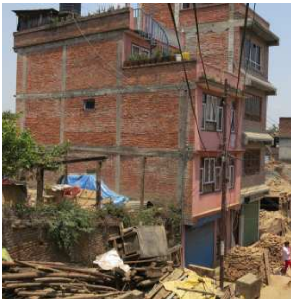
Figure 11. Reinforced concrete frames with masonry infill.
