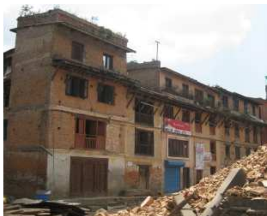
Figure 15. Urban area unconfined, unreinforced masonry buildings,
