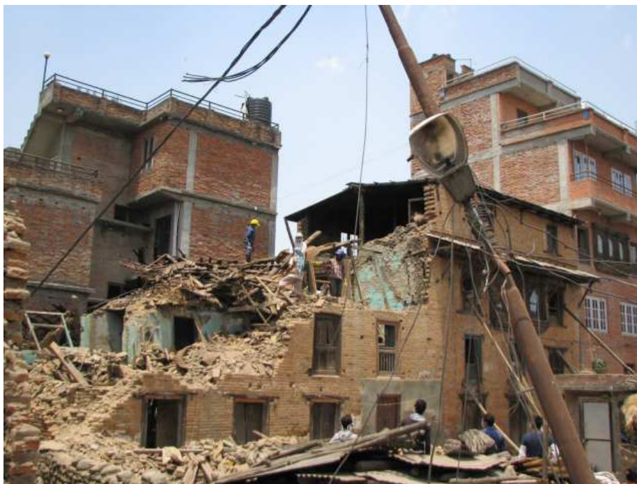
Figure 40. Unconfined masonry collapse. Note undamaged infilled frame in background, Khokana.
