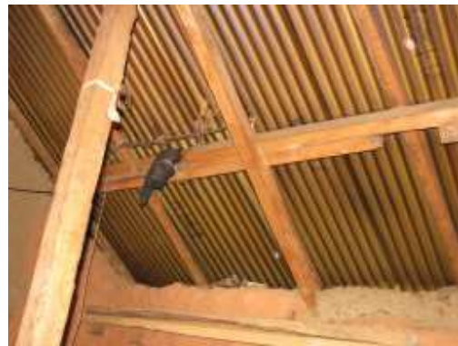
Figure 33. CGI over sloped timber roof framing, Thula Gaun.
