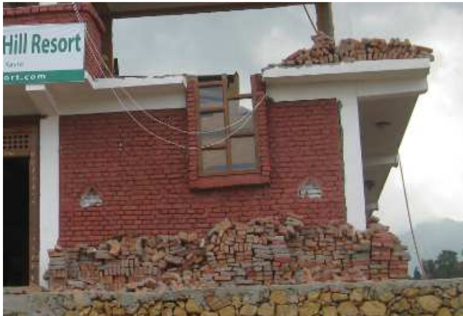
Figure 65. Construction of non-continuous, non-code complying beam at stairway of hotel structure in rural area, Thula Gaun.
