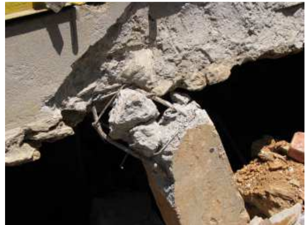
Figure 44. Foundation column failure, Chautara.
