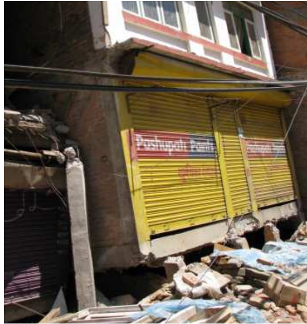
Figure 42. Foundation/lower level failure on hillside, Chautara (See Figures 43 & 44 for column failure details).
