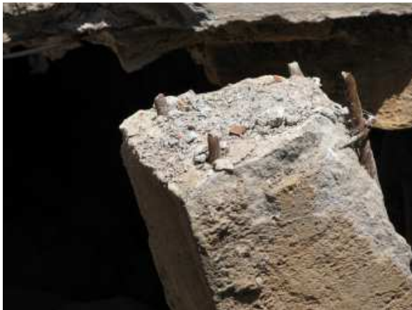
Figure 43. Foundation column failure, Chautara.
