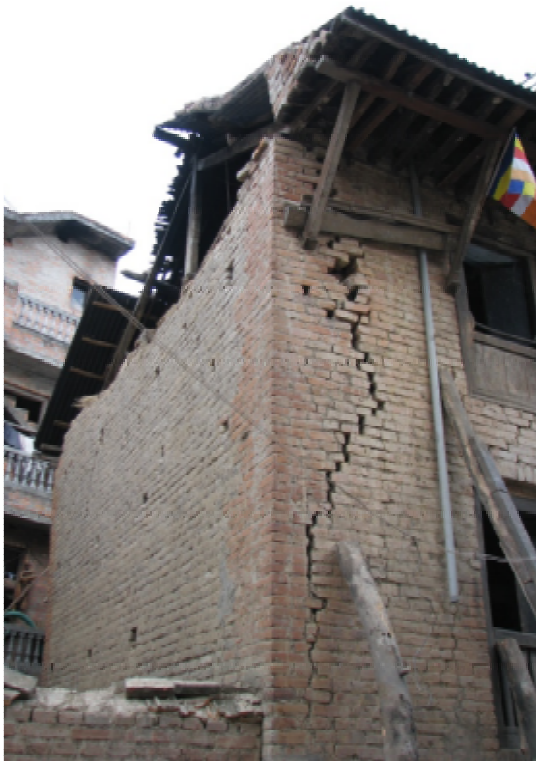
Figure 37. Gable wall failure & corner separation, Khokana.
