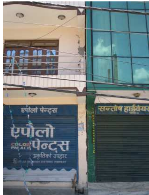
Figure 48. Pounding damage, Chautara.
