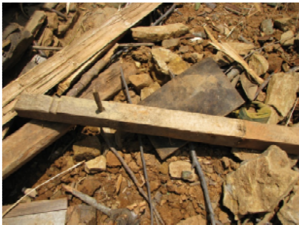
Figure 31. Pegged rafter in rubble pile, Thula Gaun.
