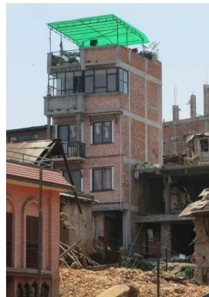
Figure 12. Reinforced concrete frames with masonry infill.
