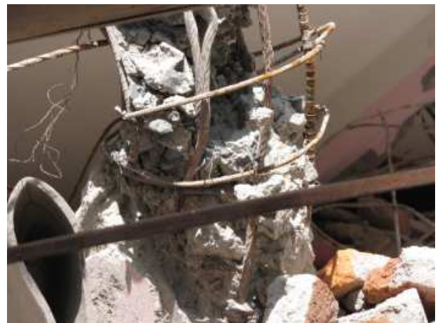
Figure 36. Close up of Figure 35 column failure, Balkhu.
