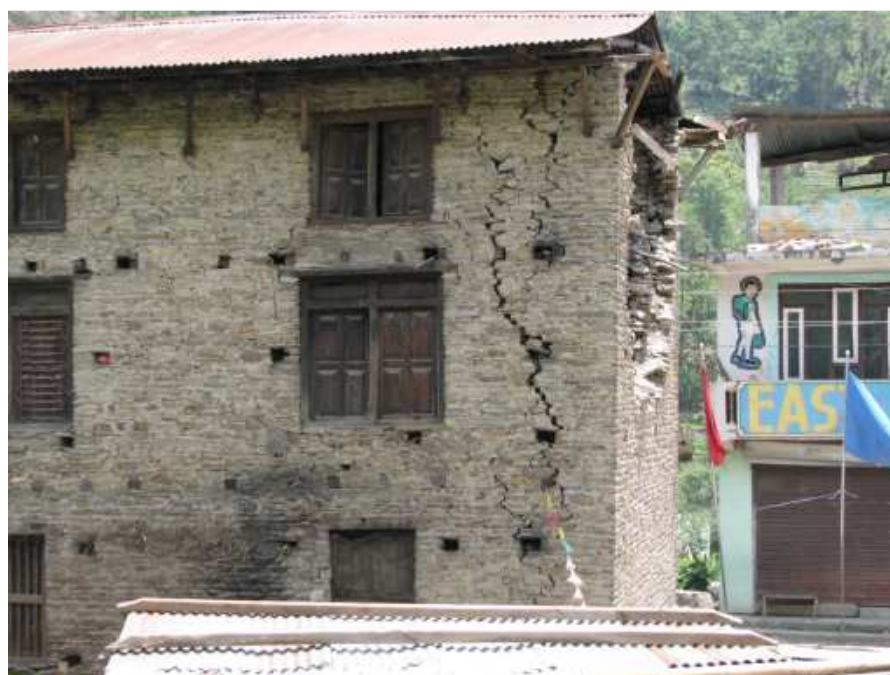
Figure 54. Damaged stone masonry with small cut stones, Mahankal.
