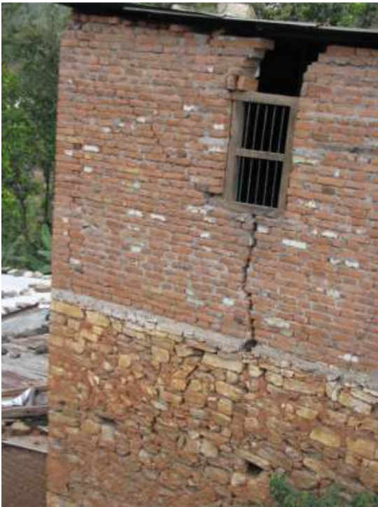
Figure 16. Brick above stone masonry, Balthali VDC.
