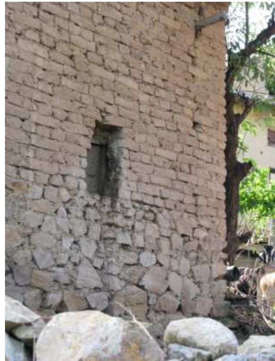
Figure 17. Brick above stone masonry, Zero Kilo.
