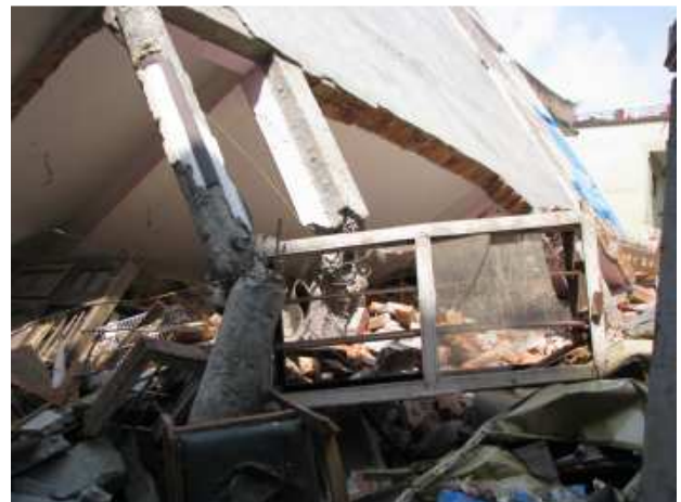
Figure 35. First story column failure, Balkhu.
