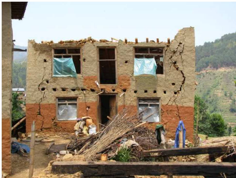
Figure 53. Severely damaged stone masonry home with randomly shaped rocks, Thula Gaun.
