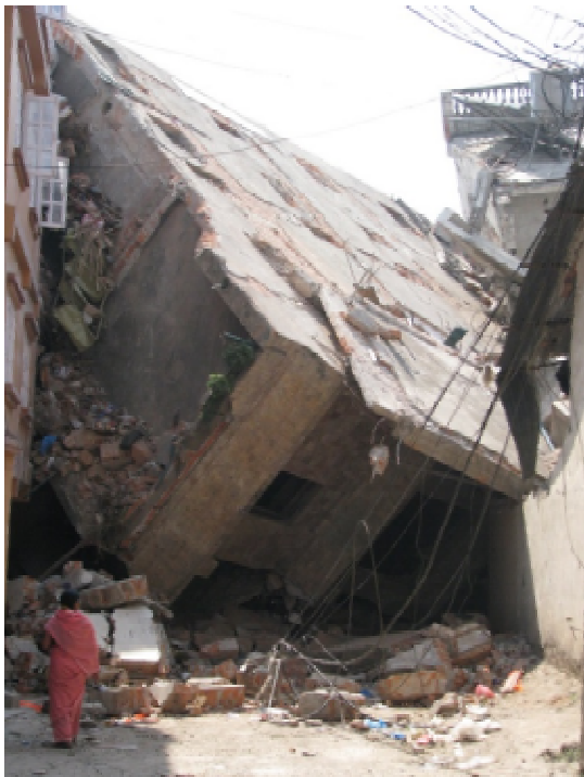
Figure 34. Soft story failure, Kuleswor.
