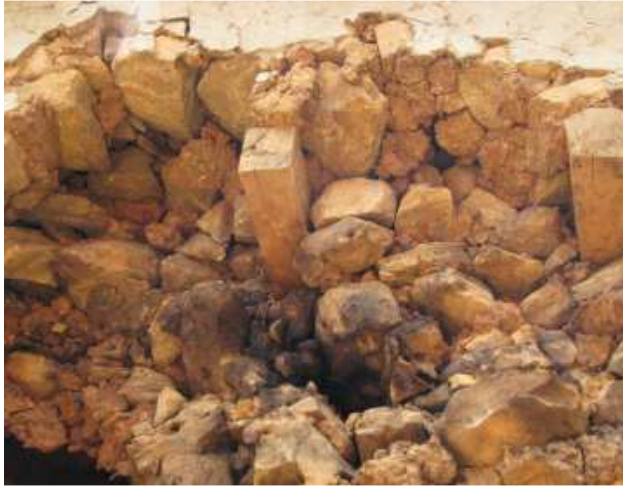
Figure 19. Random shaped stone masonry, Thula Gaun.
