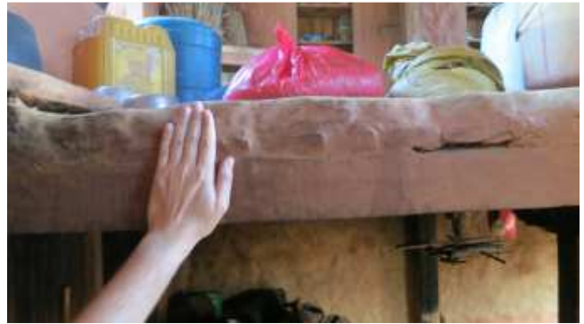
Figure 32. Mud floor over straight sheathed subfloor.
