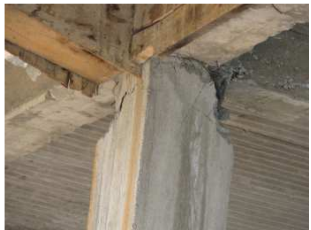
Figure 63. Beam-column connection damage, Ichok.
