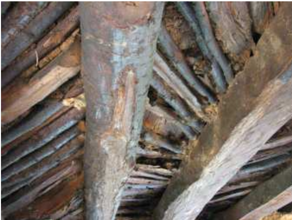
Figure 28. Herringbone subfloor layout, Thula Gaun.
