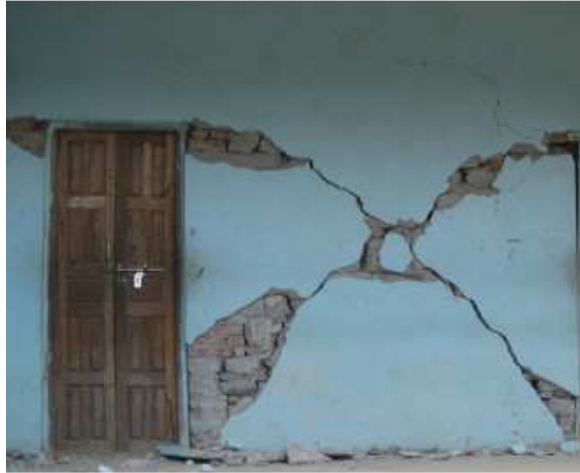
Figure 18. Use of mixed brick and stone for infill construction, to economize costs School in Mahankal.
