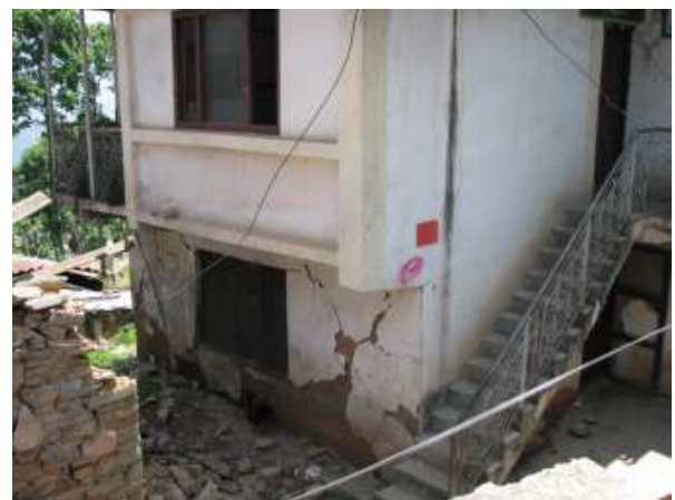
Figure 51. Red tagged structure with placard, Chautara.
