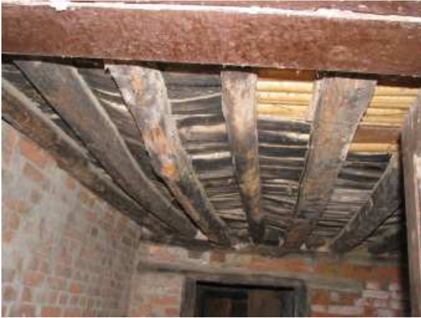
Figure 26. Example of subfloor framing, Bungamati.
