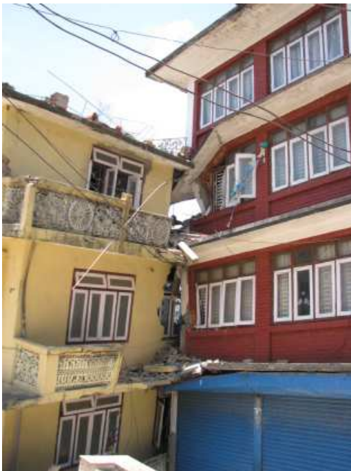
Figure 47. Damage due to adjacent building collapse, Chautara.
