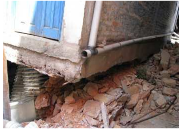
Figure 46. Foundation failure, Chautara.
