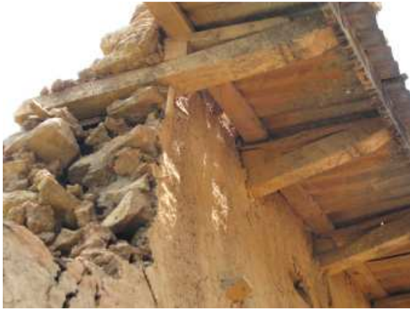
Figure 30. Pegged roof rafters in wall, Thula Gaun.
