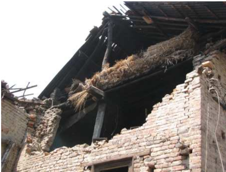
Figure 39. Collapsed end wall at gable, Bungamati.
