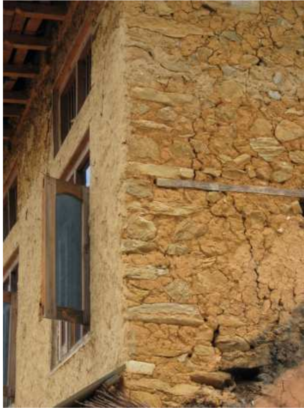
Figure 25. Example of flat cut stone with random stone shapes, Thula Gaun.
