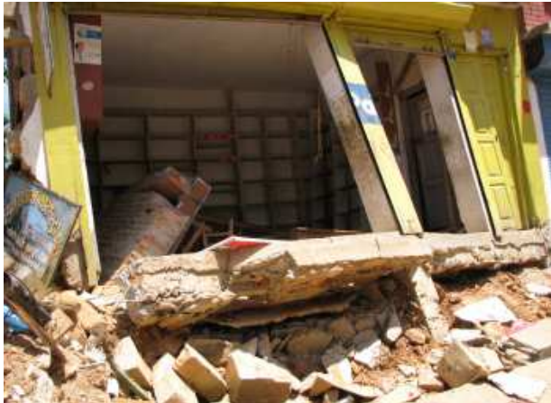
Figure 45. Foundation failure, Chautara.
