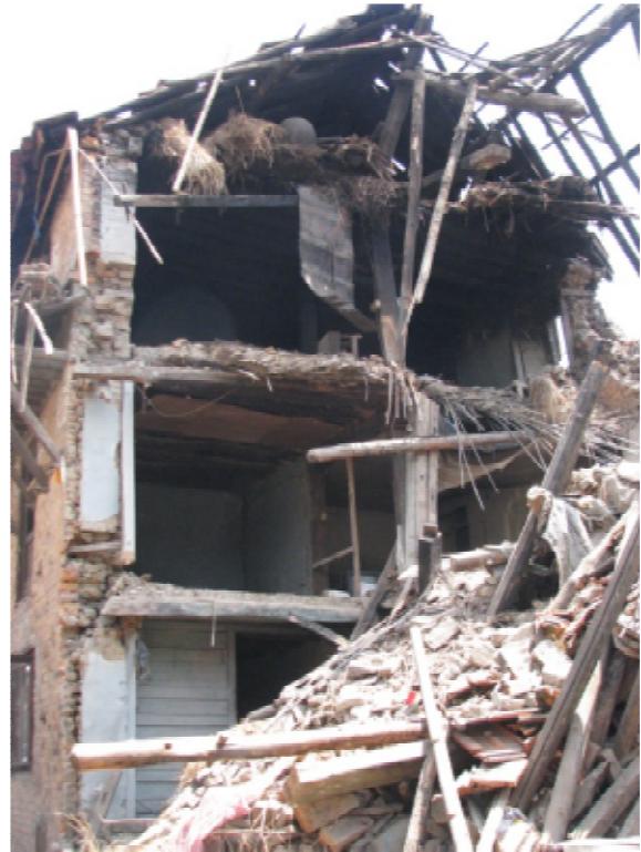
Figure 38. End wall collapse, Bungamati.
