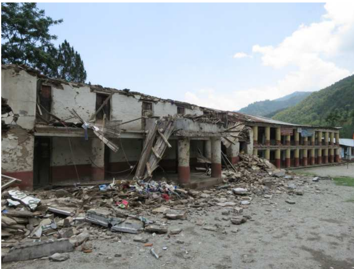
Figure 60. Heavily damaged structures, 50 and 35 years old (left to right), at Shree Saraswati School, Mahankal.
