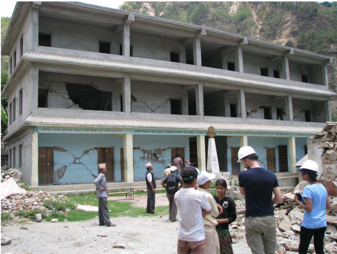
Figure 57. 3-story concrete frame Shree Saraswati School structure with shear cracking at infill walls, Mahankal.
