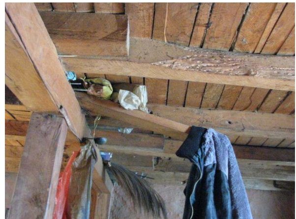
Figure 29. Straight sheathed subfloor, Thula Gaun.
