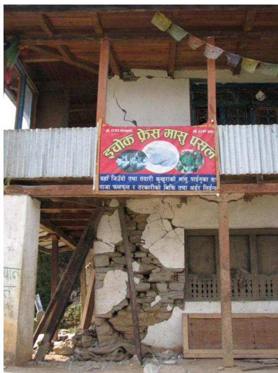
Figure 55. Large cut stones in damaged stone masonry, with plaster over stonework, Ichok.
