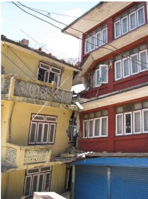
Figure 47. Damage due to adjacent building collapse, Chautara.
