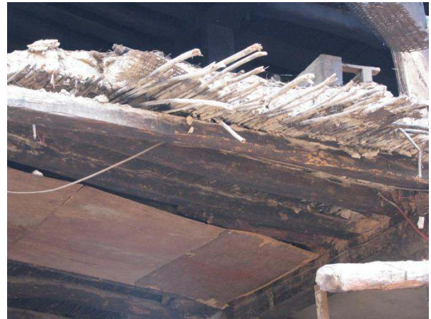
Figure 27. Example of subfloor framing, Bungamati.
