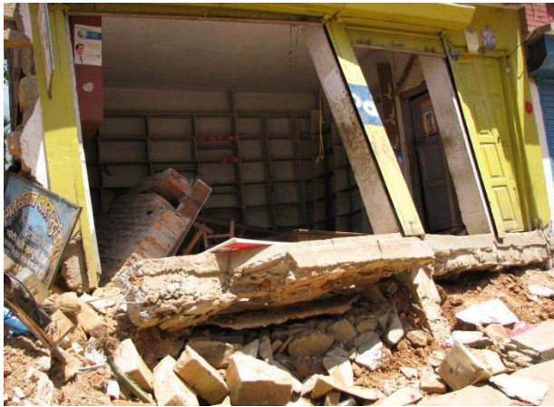
Figure 45. Foundation failure, Chautara.
