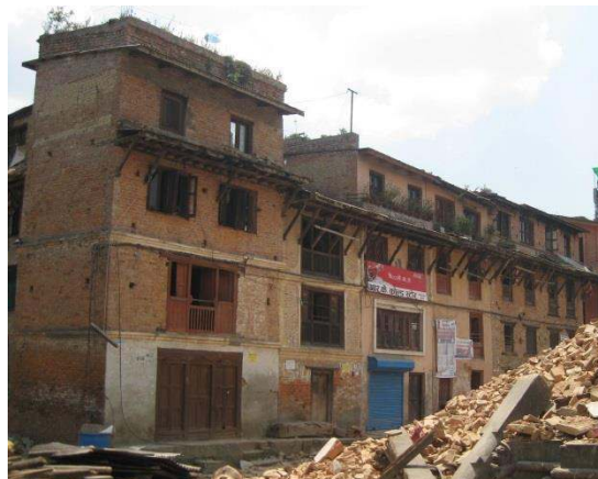
Figure 15. Urban area unconfined, unreinforced masonry buildings,
