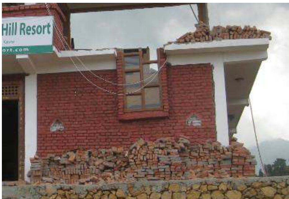
Figure 65. Construction of non-continuous, non-code complying beam at stairway of hotel structure in rural area, Thula Gaun.
