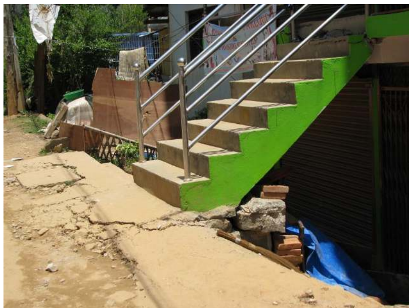
Figure 41. Evidence of foundation shifting at front of building (bottom of stair), Chautara.
