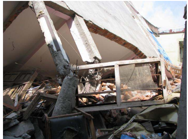
Figure 35. First story column failure, Balkhu.
