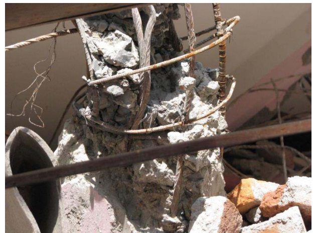
Figure 36. Close up of Figure 35 column failure, Balkhu.
