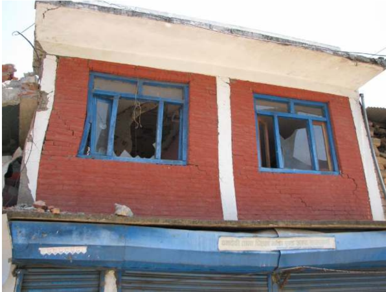
Figure 49. Damage due to pounding and collapse of adjacent building, Chautara.
