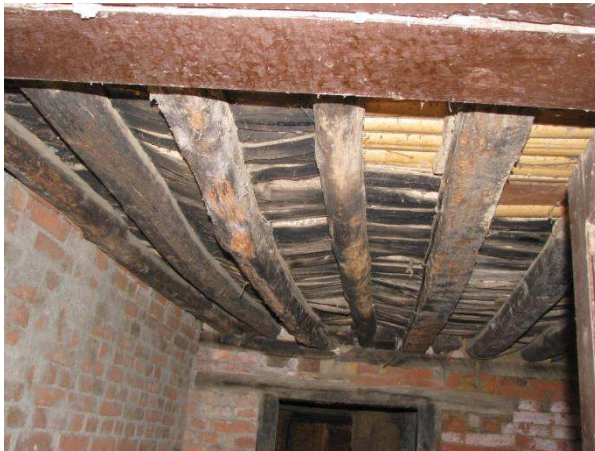
Figure 26. Example of subfloor framing, Bungamati.
