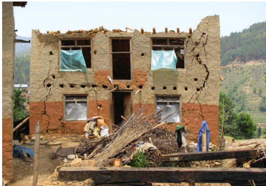
Figure 53. Severely damaged stone masonry home with randomly shaped rocks, Thula Gaun.
