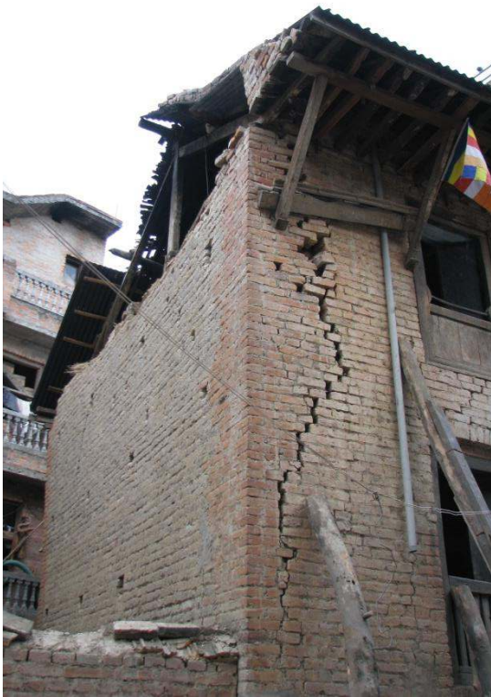
Figure 37. Gable wall failure & corner separation, Khokana.
