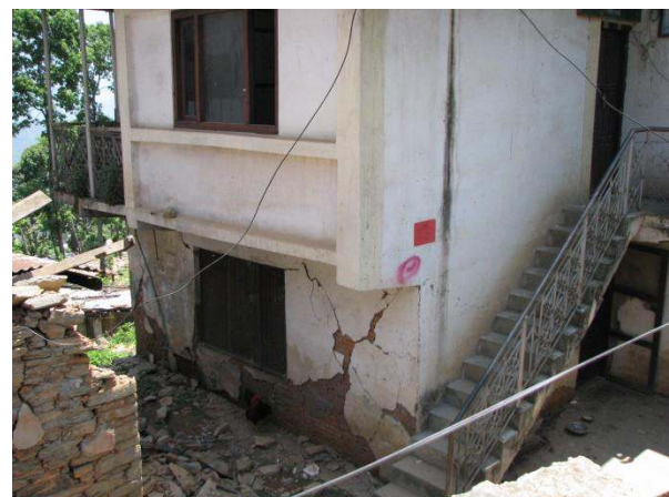
Figure 51. Red tagged structure with placard, Chautara.
