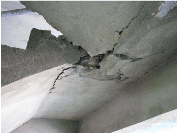
Figure 58. Concrete cracking at stair floor landing.
