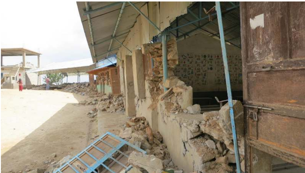
Figure 61. Damaged single-story structures at school, Ichok.
