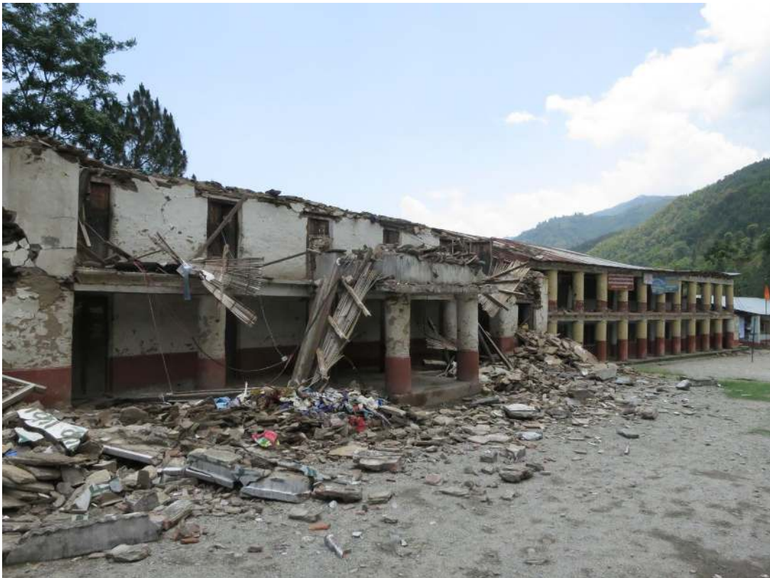
Figure 60. Heavily damaged structures, 50 and 35 years old (left to right), at Shree Saraswati School, Mahankal.
