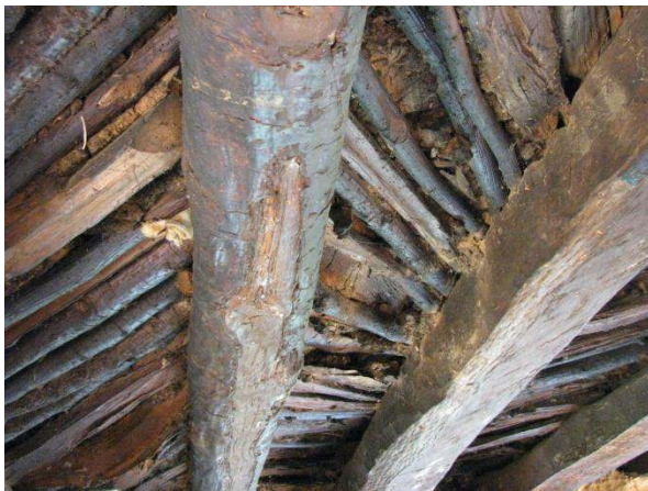
Figure 28. Herringbone subfloor layout, Thula Gaun.
