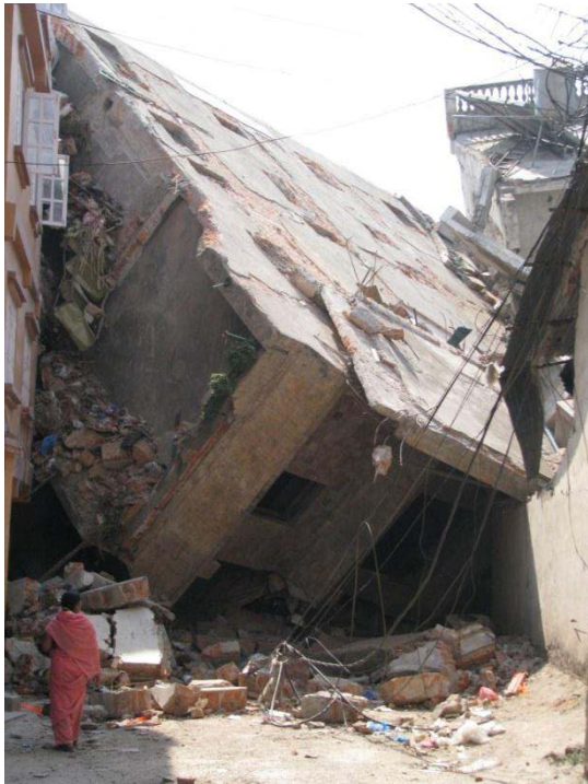
Figure 34. Soft story failure, Kuleswor.
