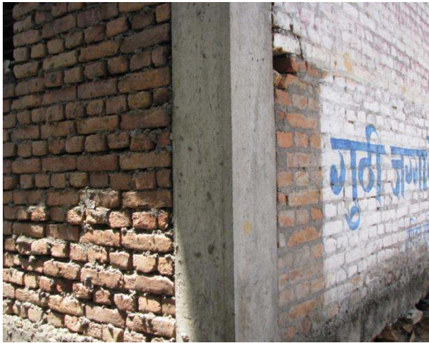
Figure 13. Note mortar finishing on exposed side wall versus mortar finish on “out of sight” back wall, Chautara.
