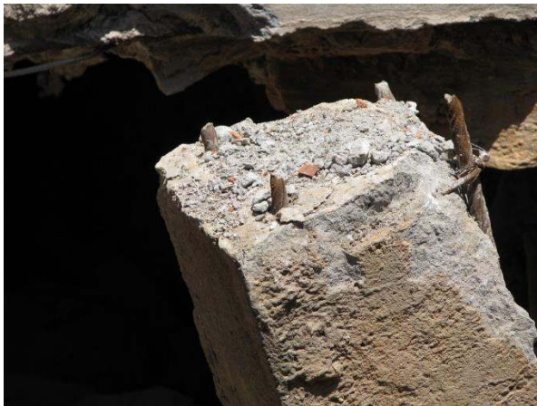
Figure 43. Foundation column failure, Chautara.
