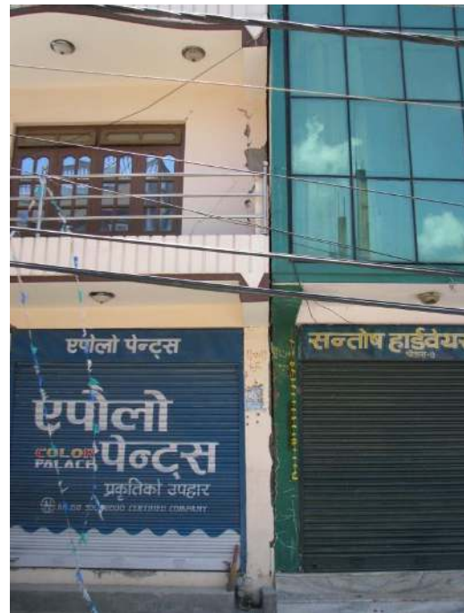
Figure 48. Pounding damage, Chautara.
