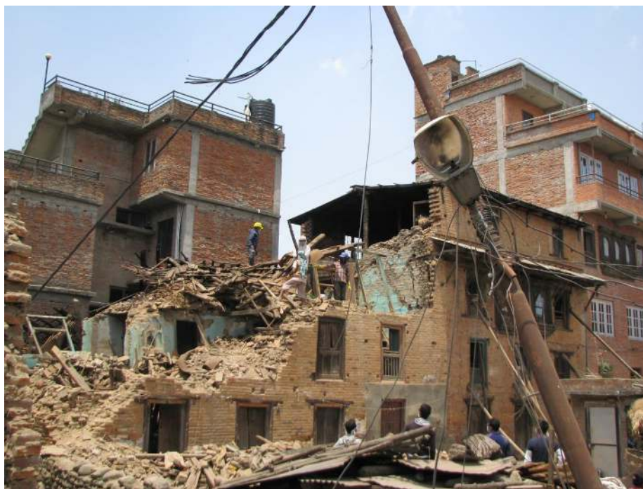
Figure 40. Unconfined masonry collapse. Note undamaged infilled frame in background, Khokana.
