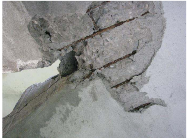
Figure 59. Close-up of stair landing spalling, Mahankal.
