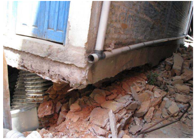
Figure 46. Foundation failure, Chautara.
