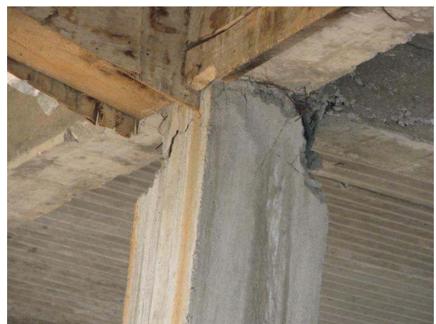
Figure 63. Beam-column connection damage, Ichok.
