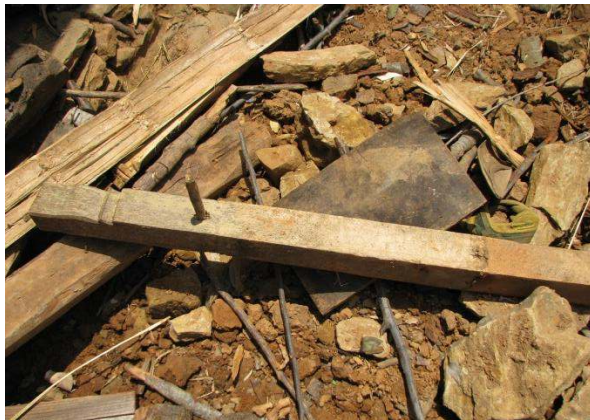
Figure 31. Pegged rafter in rubble pile, Thula Gaun.
