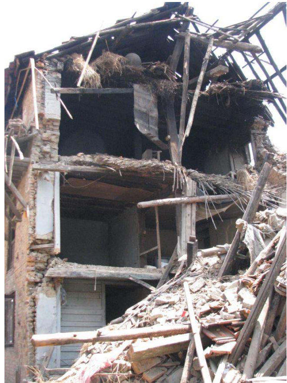
Figure 38. End wall collapse, Bungamati.
