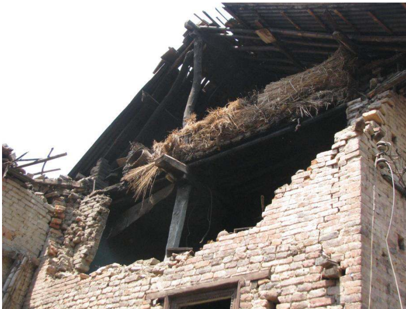
Figure 39. Collapsed end wall at gable, Bungamati.
