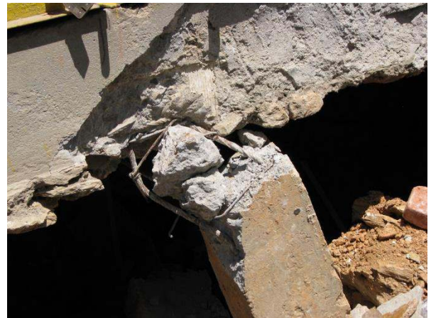
Figure 44. Foundation column failure, Chautara.
