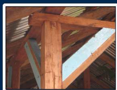
Diagonal bracing in all 4 corners
