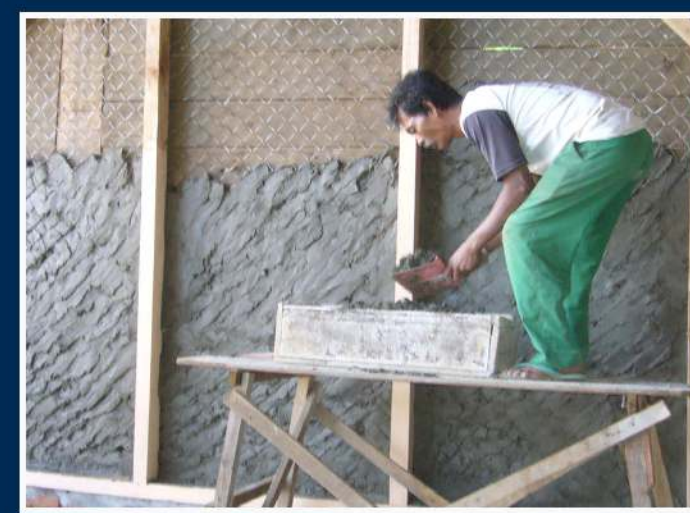
Install backing boards and plaster
