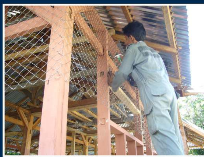
Install the chain-link lath and bend nails over to stretch it tightly
