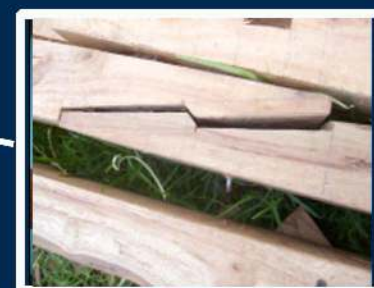
Use proper splice joinery
