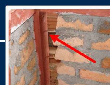
The masonry skirt may be made from bricks or concrete blocks but it must have a nail connecting masonry to column
