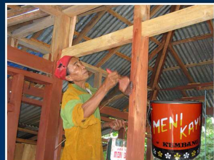
Before plastering, be sure to paint all timber with preservative paint
