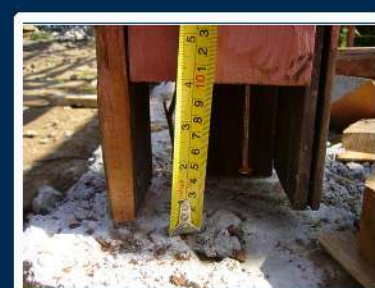
Keep wood column off ground with concrete starter
