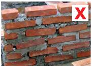
4. 错开竖缝且不要使用坏砖 Stagger vertical joints and do not use broken or half bricks
