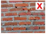
3. 灰缝厚度应是0.8cm到1.2cm, 厚度要一致 Joint spacing between bricks should be consistent and between 0.8cm and 1.2cm
