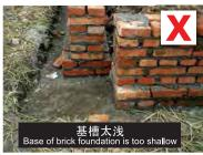
基槽深度按土质决定,推荐砖基 础底部离地面不少于50cm。最低 要求基础总埋深不少于50cm。 Depth of foundation trench depends on soil strength, but the base of the brick foundation should be at least 50cm below the ground surface. The minimum requirement for the
