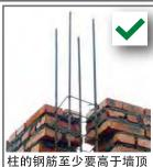
0.56m, 用于搭接上圈梁 Steel reinforcement in the tie column should extend at
