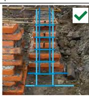
在构造柱处, 砌砖基础应建有马雅 槎。构造柱中钢筋应该延伸至砖基 础底部,端部弯勾长度至少36cm。 The long bars from the column should extend to the base of the foundation and terminate with anchors that are at least 36cm long
