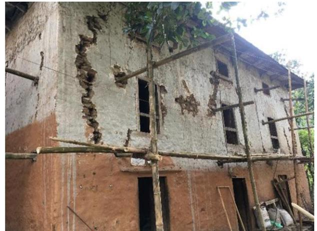
Fig. 26. Damaged house prior to retrofitting
