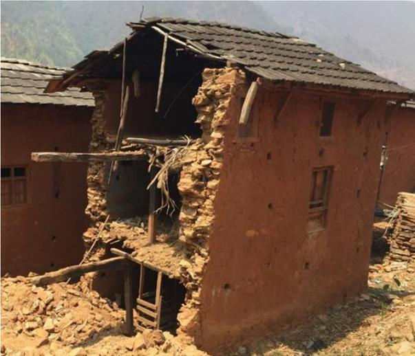
Fig. 11. A damaged house in Sindhupalchowk where the entire short wall is collapsed but the house is still standing
