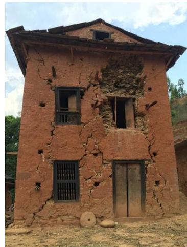
Fig. 9. Short wall damage
