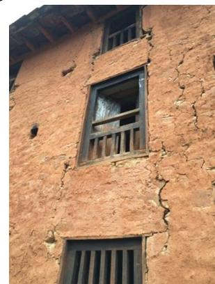
Fig. 10. Vertical cracks observed at floor level in a typical SMM house
