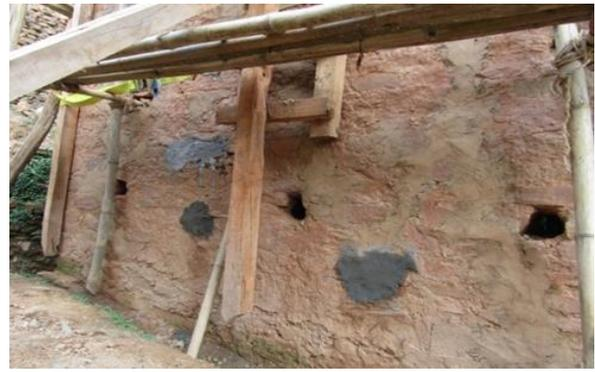
Fig. 13. Installed through wall concrete connections
