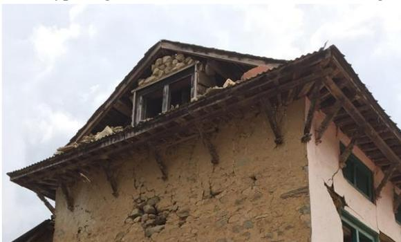
Fig. 8. Gable wall damage after earthquake
