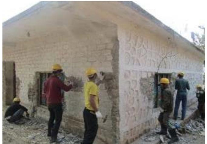
Figure 20: Trainee masons working on removal of cement plaster and surface preparation of house undergoing retrofitting
