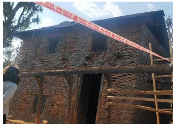
**Figure 17: Retrofit of a house using splint and bandage approach**
