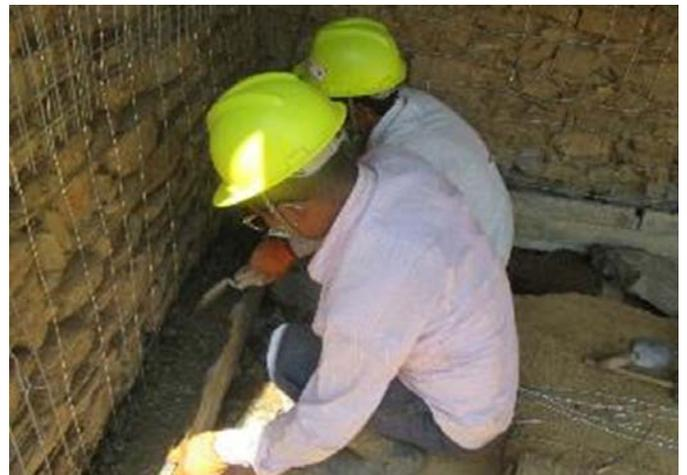
Figure 26: Concreting of foundation tie beam after completion and anchorage of reinforcements
