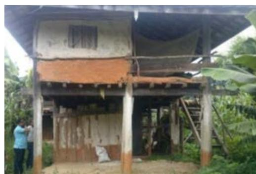
Figure 5: Typical timber frame structure
