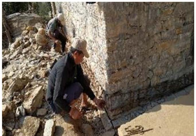
Figure 22: Mason preparing foundation for lateral tie beam below the plinth level for tying up reinforcements
