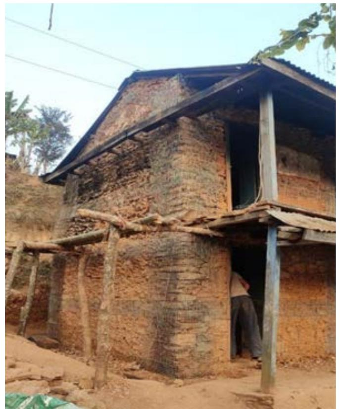
Figure 30: Securing “splints” vertically at critical junctions of the walls
