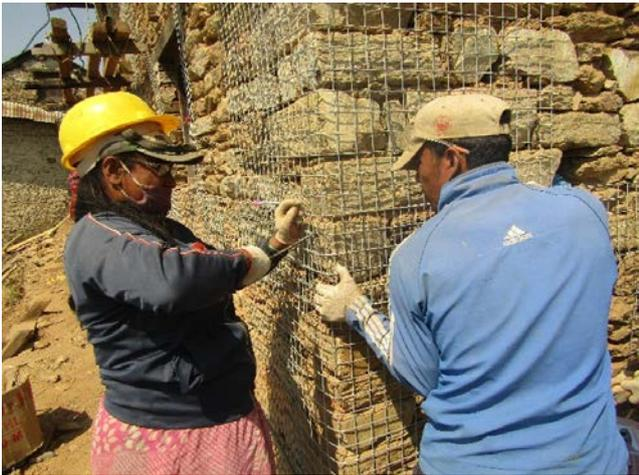
Figure 23: A pair of masons fixing vertical and horizontal strips of welded GI wire mesh as splints and bandages during retrofitting in Dolakha
