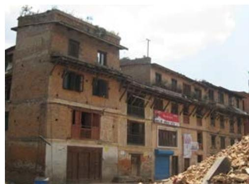
**Figure 3: Typical brick in mud mortar house**
