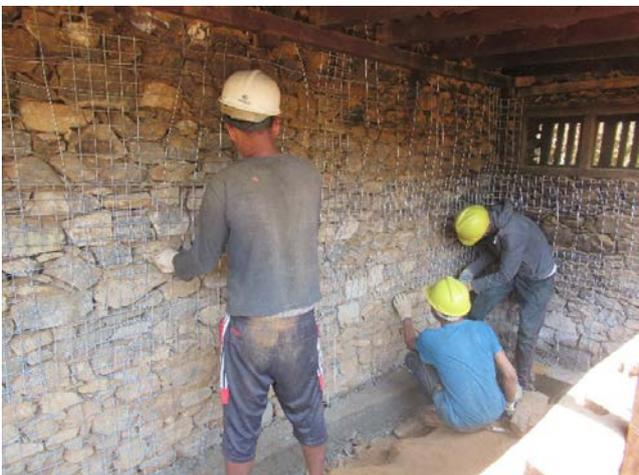
Figure 25: Preparing wire mesh using GI wires and anchoring to the wall to prevent local failure in stone masonry building
