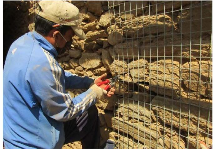
Figure 24: Anchoring inner and outer mesh of GI wires
