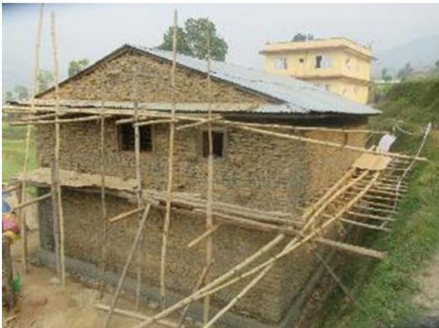
Figure 19: Scaffolding and props seen around a stone-mud masonry house undergoing retrofitting in Nuwakot
