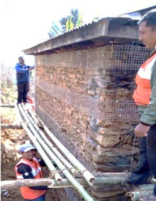
Figure 29: Securing the “bandages” horizontally on walls
