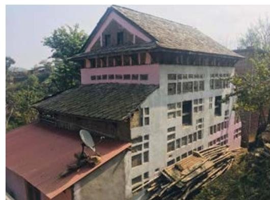
**Figure 28: Example of CR integrated splint and bandage technology**
