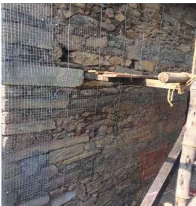
Figure 31: Containment reinforcement wires (vertical & horizontal) put in place
