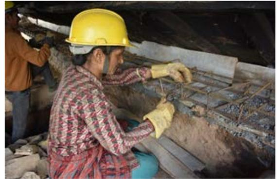
**Figure 52: Participant constructing ring beam at ongoing training on strong back**
