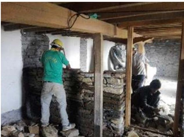
Figure 21: Ongoing architectural modification work on construction of wing walls during retrofitting of house in Dolakha
