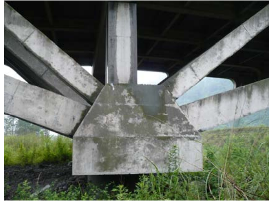
Fig 17. Spandrel supports, between 1 st and 2 nd spans from the east. IMG0033
