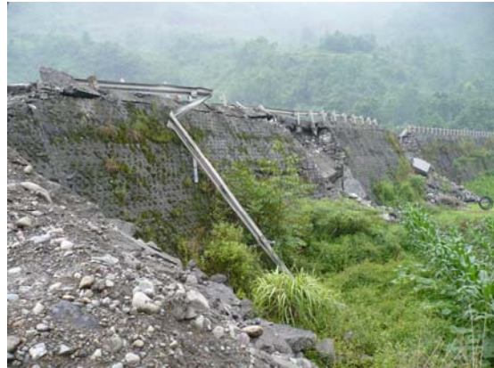
Fig 7. South side of east approach, looking ENE. IMG0015
