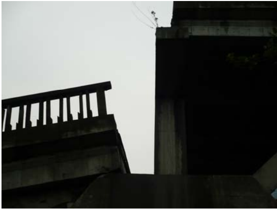
Fig 18. Collapsed deck in 3 rd span (shown at left). IMG0037
