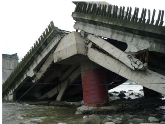
Fig 23. Pier between 3 rd and 4 th spans, not clear if pier displacement caused the collapse, or the pier was pushed west by the collapsing deck. IMG0048
