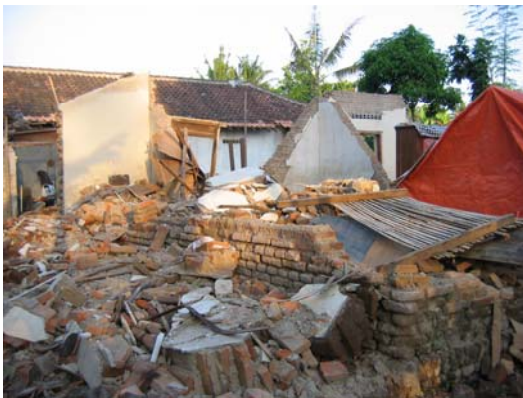
Figure 4. Destroyed unreinforced masonry houses, Pleret (Bantul), S7.83686° E110.41552° IMG_6633
