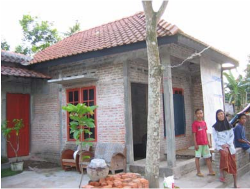
Figure 8. Well designed and built confined brick masonry house, edge of heavily damaged Pleret (Bantul), S7.83686° E110.41552°, IMG_6636
