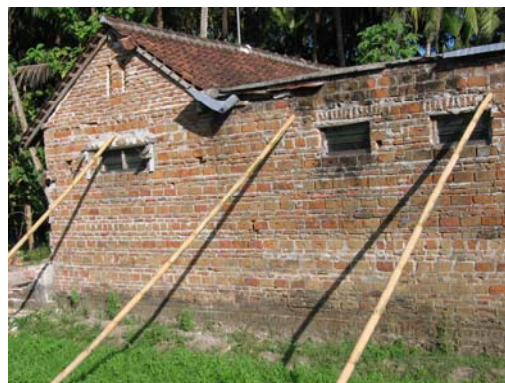
Figure 7. Unreinforced masonry, Bebekan Mulyodadi, Bambang Lipuro (Bantul). S7.94160°, E110.32297° IMG_6806
