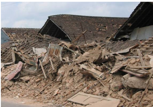
Figure 2. Debris along main street through Imogiri, S7.92282°, E110.38374° IMG_6551
