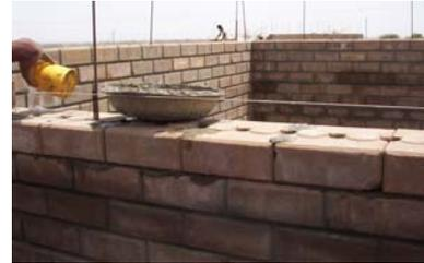
Fig. 10. Interlocking compressed stabilized earth wall
