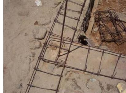
Fig. 6. Reinforcement for plinth band
