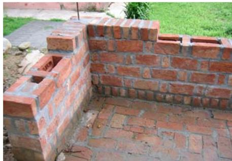
Fig. 8. Brick masonry using rat-trap bond
